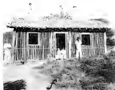
PLATE 6. House types and construction. a , House, made of pau a pique , or puddled earth spread over structure of poles and sticks; roof is of sape , a coarse grass. b , House of brick, held together with dried mud, with tile roof. c , Brick house covered with reboque (a kind of plaster) and calcimined in pink, with white trimming. d , Large farm dwelling, known as "The Casa Grande"; walls are of taipa , or tamped earth, about 2 feet thick; roof is of tile. e , Three houses with a common front and roof; windows and doors are of unpainted boards. f , Framework of a pau a pique house. g , Covering framework of f with puddled earth. h , Pau a pique wall after drying.
