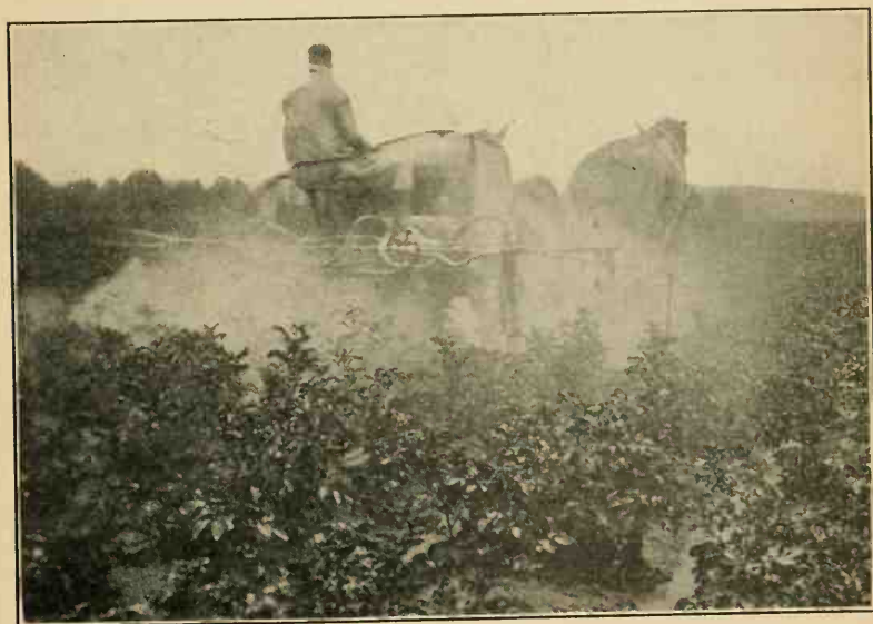
FIG. 2—SPRAYING UNDER HIGH PRESSURE PRODUCES A VERY FINE MIST With three nozzles per row, it is possible to apply 100 gallons of Bordeaux mixture per acre.
