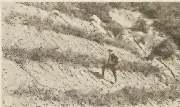
FIGURE 8.—SECTIONS OF FILL SLOPES ABOUT 70 FEET BELOW GRADE. A; EROSION ON AN UNPROTECTED FILL. B; A FILL PROTECTED ACCORDING TO METHOD A.
