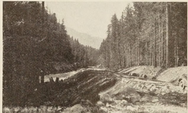
FIGURE 3.—A COMPLETED CHANNEL CHANGE THAT DIVERTS THE STREAM FROM ITS ORIGINAL CHANNEL ENTIRELY.
