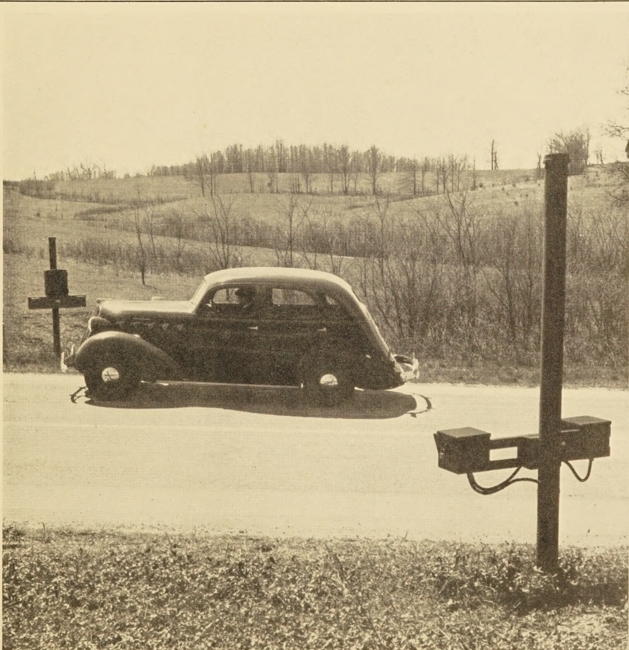
AUTOMATIC TRAFFIC RECORDER INSTALLED ON U S 240 IN MARYLAND
