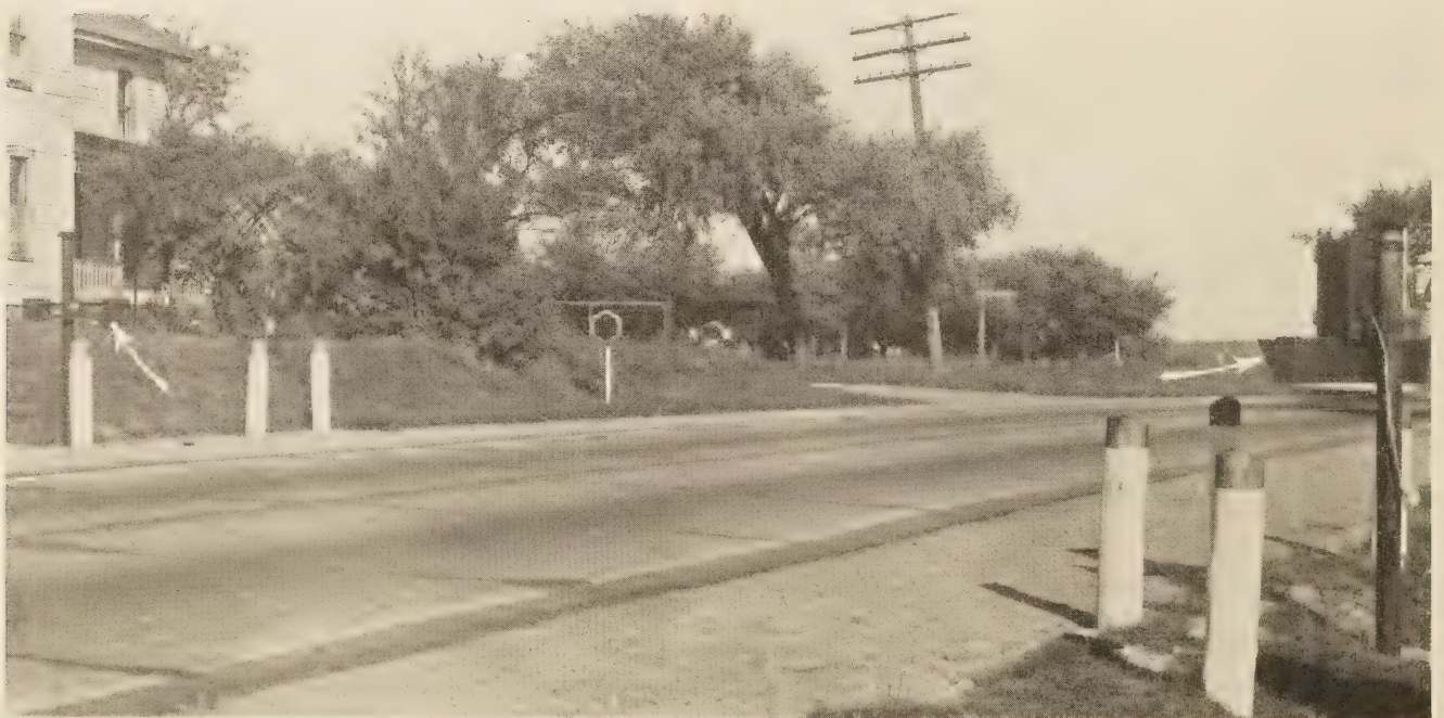
FIGURE 6.—AUTOMATIC TRAFFIC RECORDER INSTALLATION IN MICHIGAN. NOTE GUARD POSTS TO PROTECT RECORDER FROM TRAFFIC.
