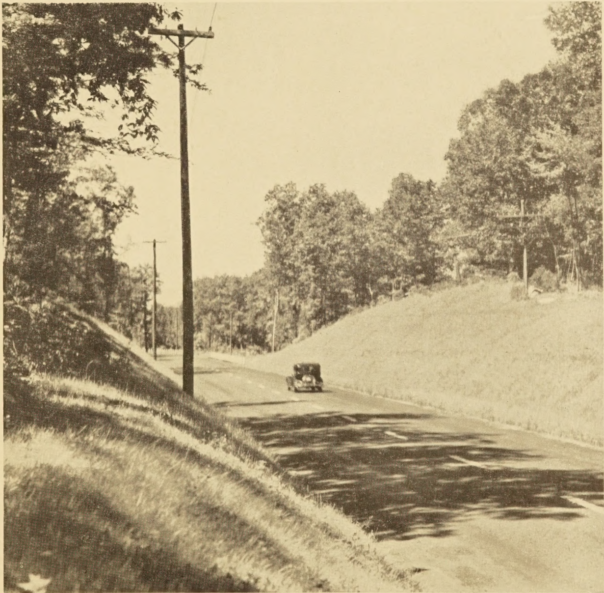
ROUNDED CUT SLOPES ON A CONNECTICUT HIGHWAY
