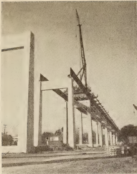
Construction under way on the Jacksonville Expressway in Florida.
