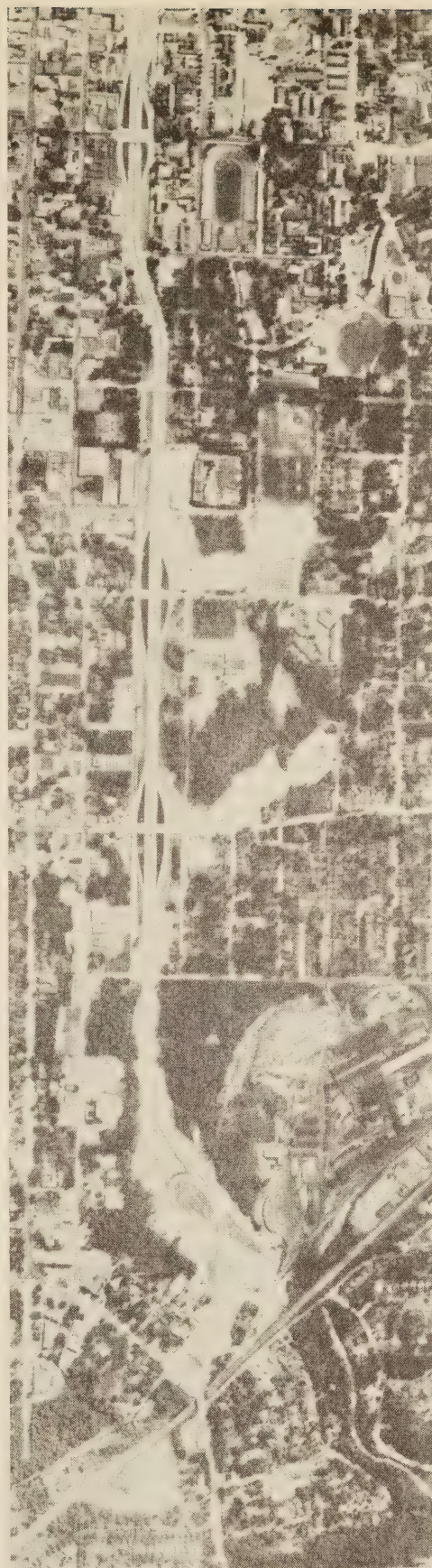
The Atlanta Expressway, Georgia.
