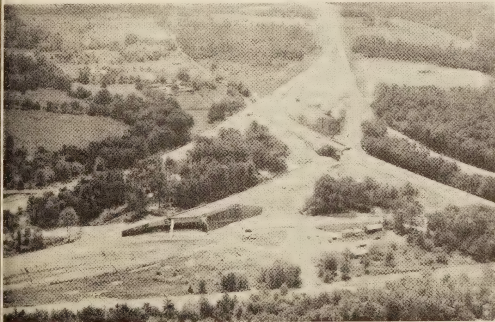
Construction of the airport interchange in Maryland: Baltimore-Washington Expressway.
