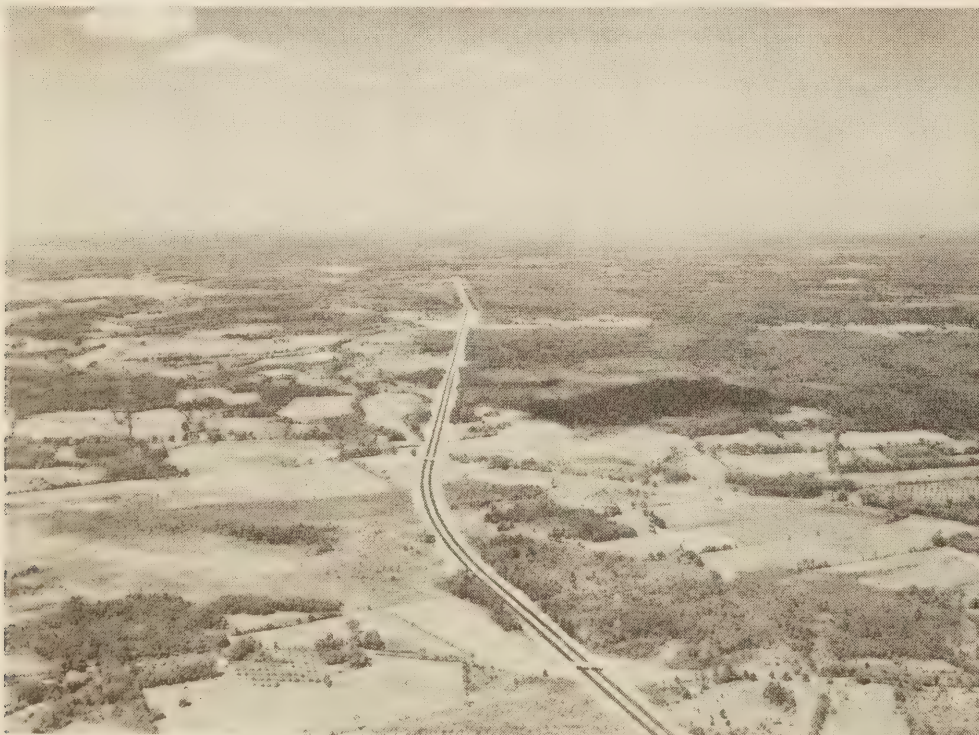
The New Hampshire Turnpike.
