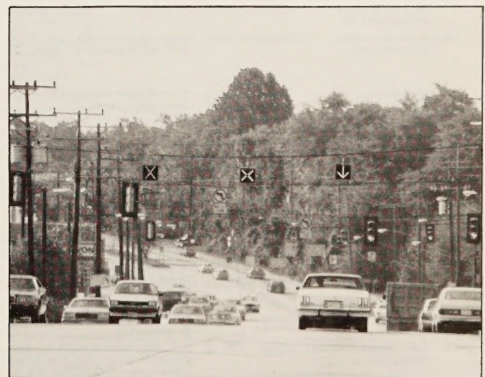
Figure 7. — Lane-use signals — Montgomery County, MD.
