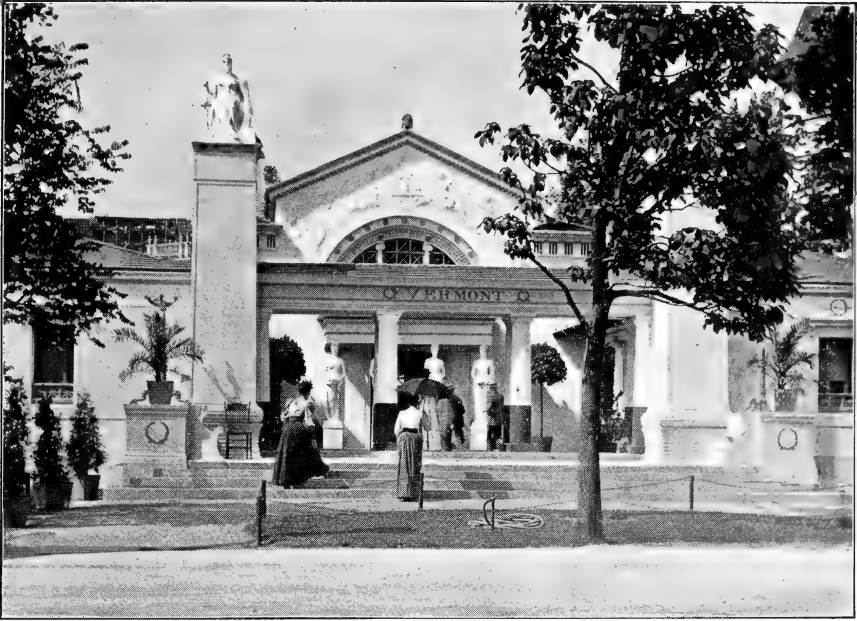
THE VERMONT STATE BUILDING.
