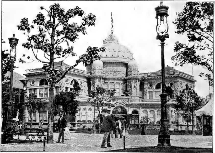
THE MISSOURI STATE BUILDING.
