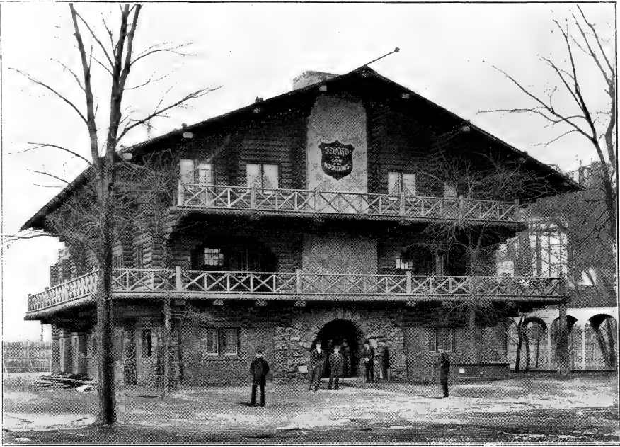
THE IDAHO STATE BUILDING.
