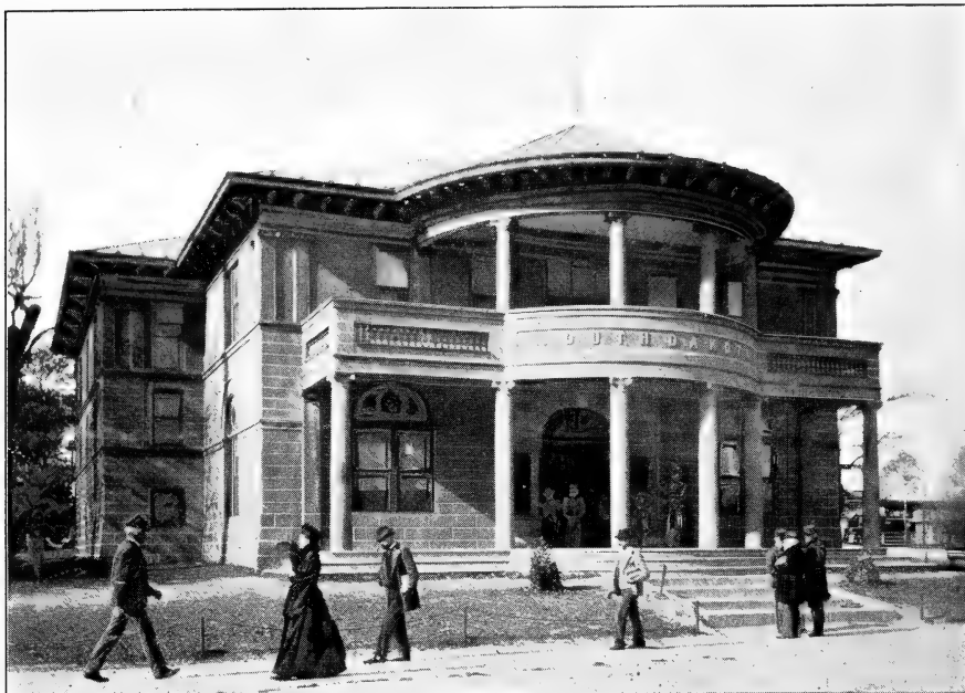
THE SOUTH DAKOTA STATE BUILDING.
