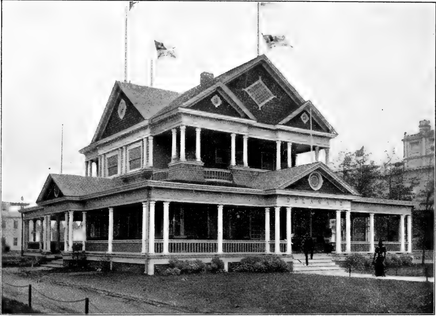
THE DELAWARE STATE BUILDING.
