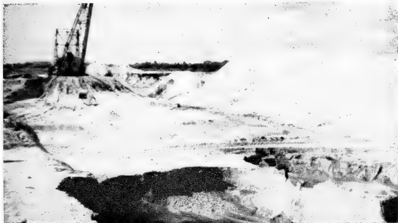
Figure 3.—The matrix (ore) of pebble phosphate in foreground with overburden removed.
