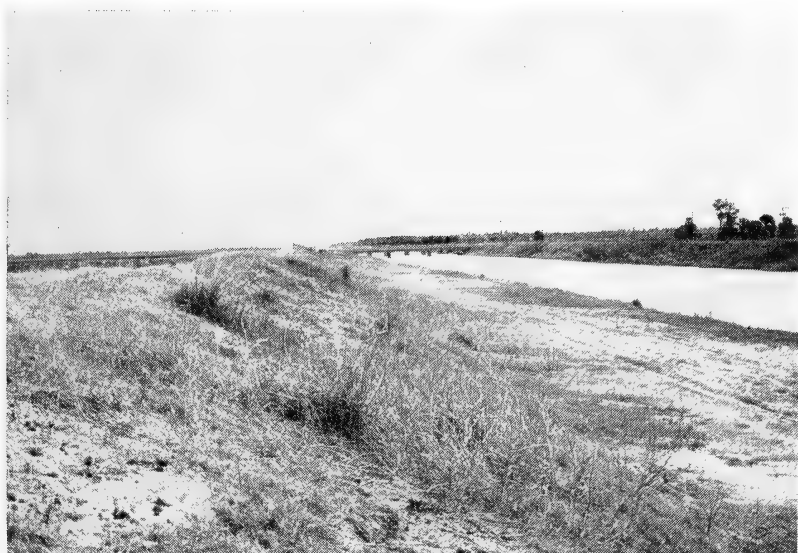
Fig. 1. View of Rim Ditch Canal looking southeast toward the Florida East Coast Railroad bridge.
