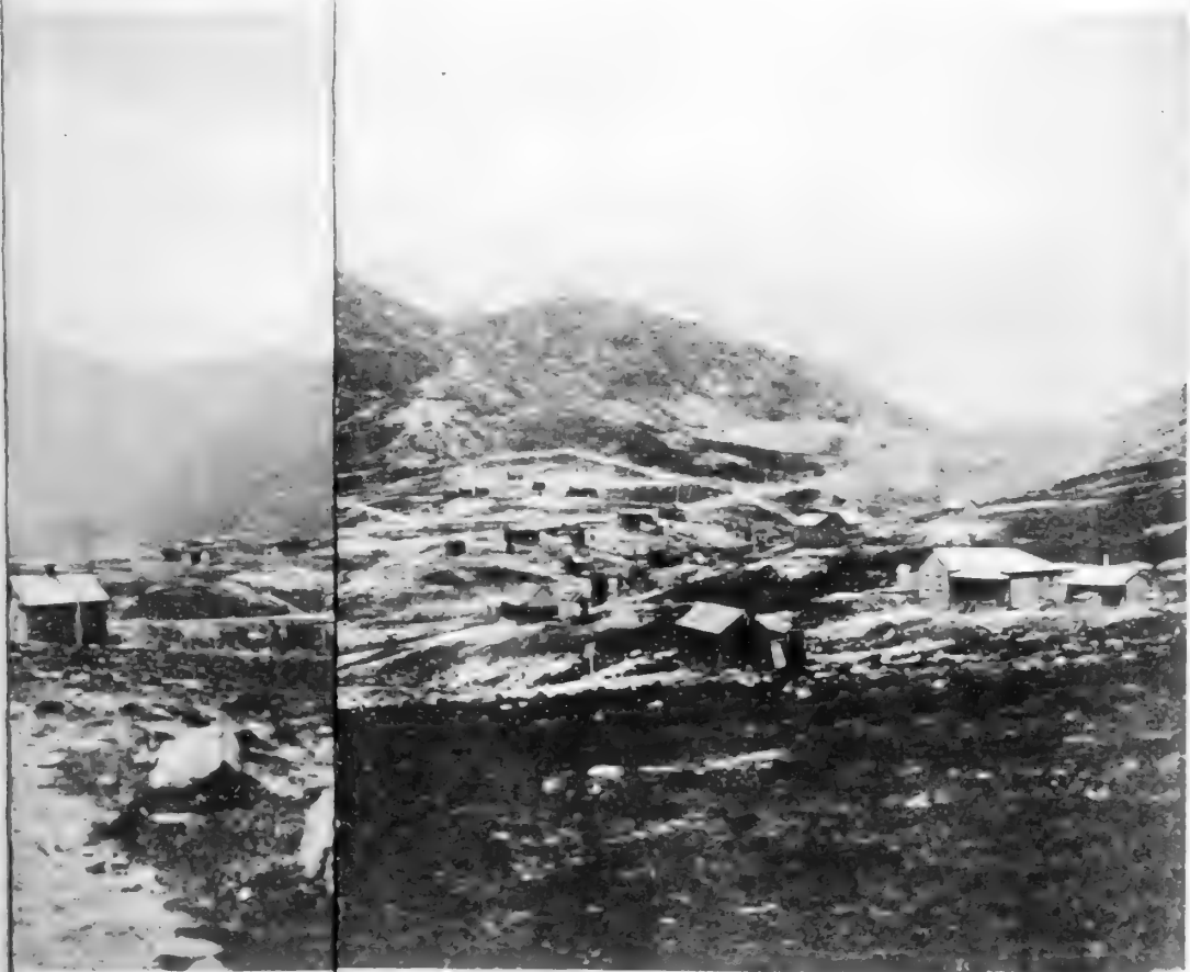
OWEN, THE GORMANMOUNT-LYELL MINE OFFICES.
