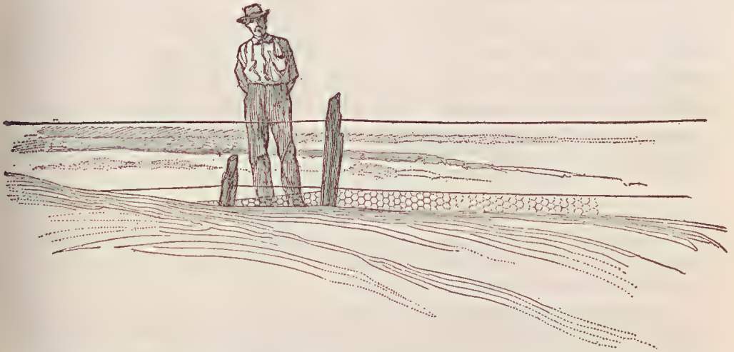
COBHAM LAKE HORSE Paddock.—NETTING FENCE COVERED BY DRIFT-SAND, AND NEW ONE ABOVE.
