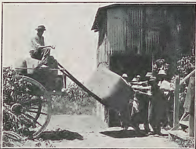
PLATE 39 (FIG. 4).—LOADING INTO RAILWAY TRUCKS AT KAMMA, NEAR CAIRNS.
