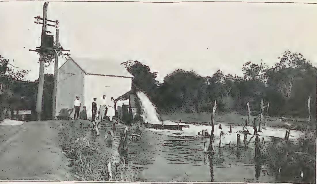
PLATE 139.—PUMPING STATION, BOWEN SALT LIMITED, BOWEN, NORTH QUEENSLAND.
