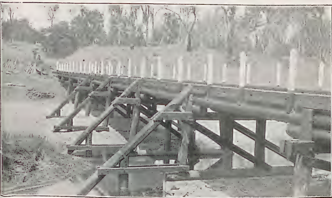
PLATE 162. LOW-LEVEL BRIDGE, STUART RIVER, WONDAL-PROSTON ROAD.
