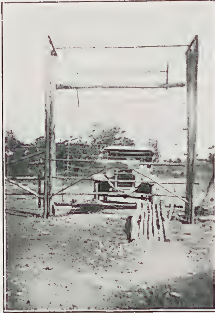
PLATE 164 (Fig. 1).—GATE DOWN; CAR APPROACHING.
