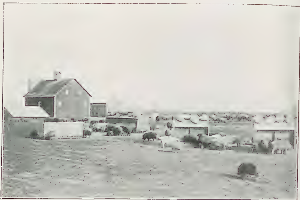
PLATE 131 (Fig. 4).—SELF-FEEDING SYSTEM IN OPERATION ON A LARGE AMERICAN PIG FARM.
