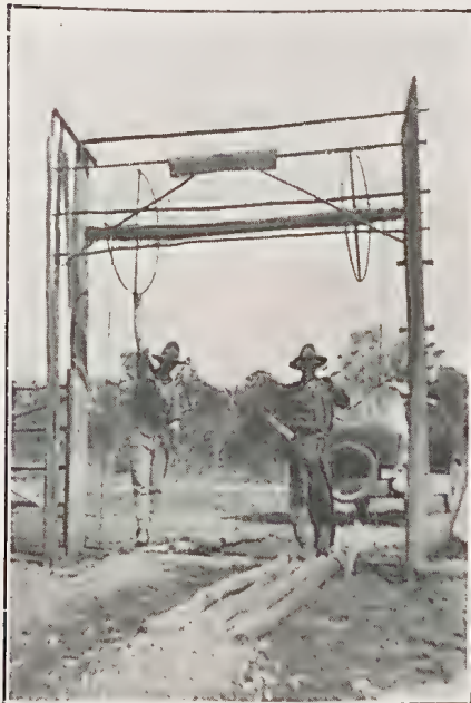
PLATE 167 (Fig. 4).—GATE RISEN BY THE WEIGHT OF TWO MEN STANDING ON BEARERS; GATE UP.
