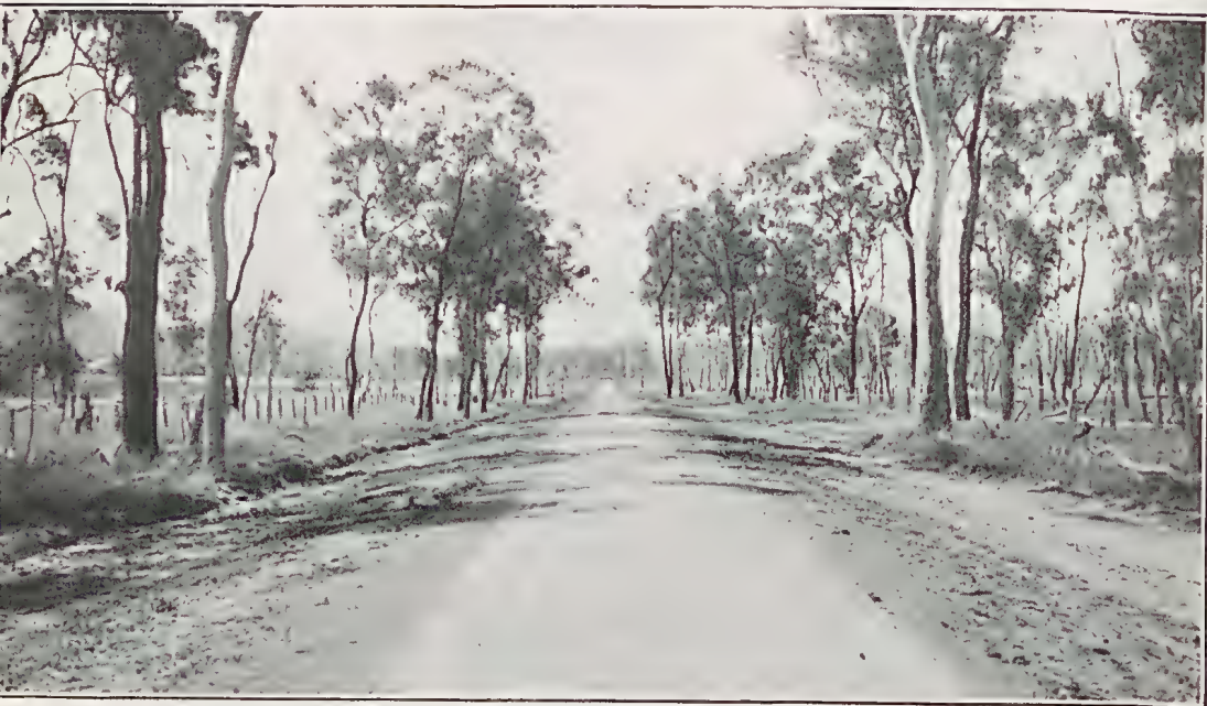
PLATE 161. "C" CLASS METAL, GOOMERI-CHILDERS ROAD, NEAR BIGGENDEN.
