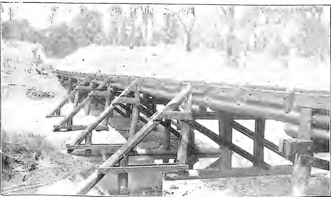
PLATE 162. LOW-LEVEL BRIDGE, STUART RIVER, WONDAL-PROSTON ROAD.
