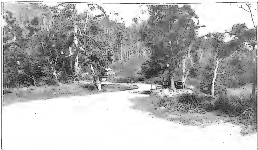
PLATE 163. CAIRNS-PORT DOUGLAS ROAD.
