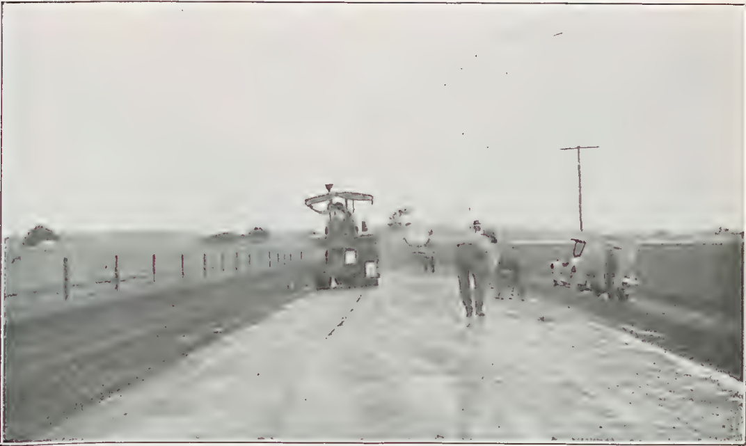
PLATE 21. ROLLING, WATERING, AND BROOMING, HARRISVILLE-ROSEVALE ROAD.
