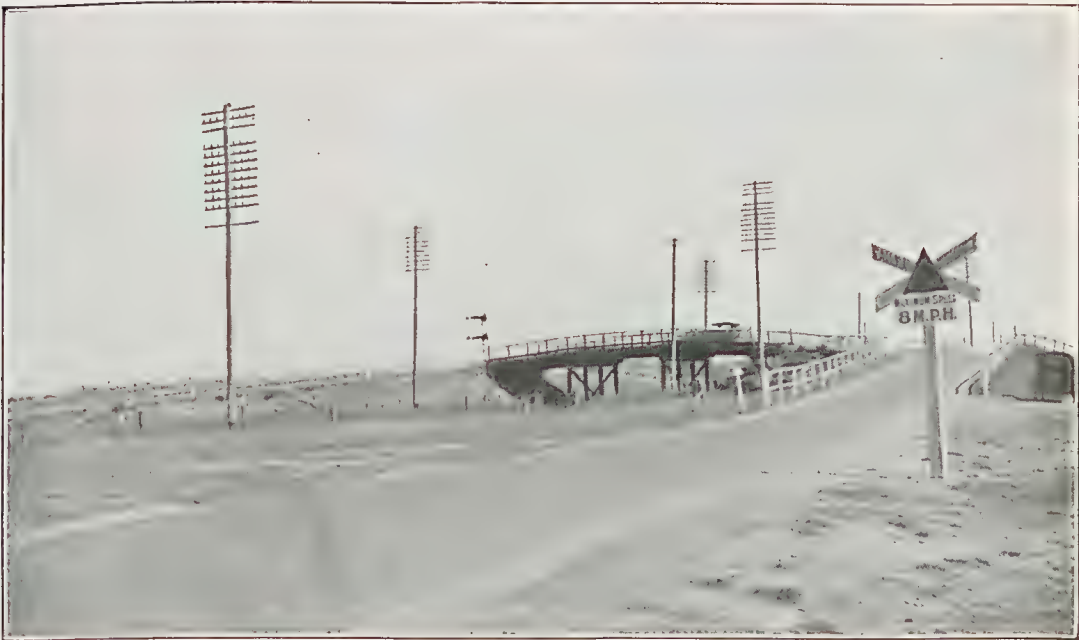
PLATE 22. IPSWICH ROAD, REDBANK, AFTER CONSTRUCTION, SHOWING CONGLOMERATE ROAD SURFACED WITH BITUMEN. STANDARD WARNING SIGN DISPLAYED.
