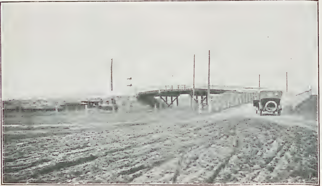
PLATE 23. IPSWICH ROAD, REDBANK, BEFORE CONSTRUCTION.
