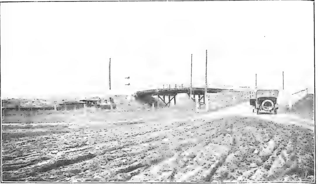
PLATE 23. IPSWICH ROAD, REDBANK, BEFORE CONSTRUCTION.
