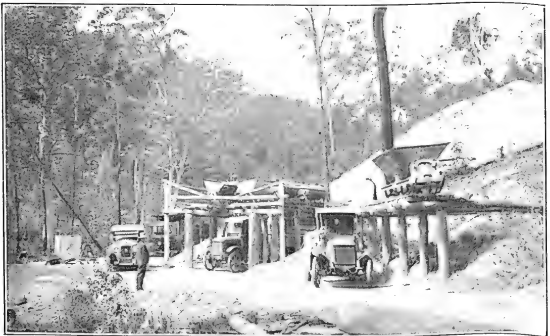
PLATE 20. DOCK LOADING FROM SIDE-TIPPING TRUCKS—CONGLOMERATE QUARRY, MAIN SOUTH COAST ROAD.
