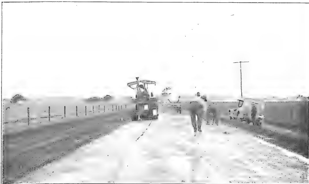
PLATE 21. ROLLING, WATERING, AND BROOMING, HARRISVILLE-ROSEVALE ROAD.
