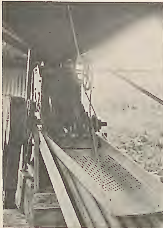
INTERIOR OF W. A. HANNAM'S PULPING-HOUSE.
