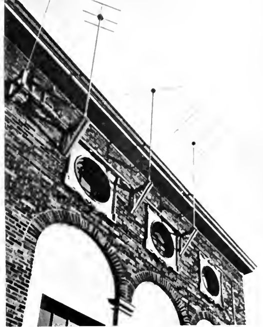
ANTENAPLEX INSTALLATION ON PARK LANE HOTEL IN NEW YORK.
