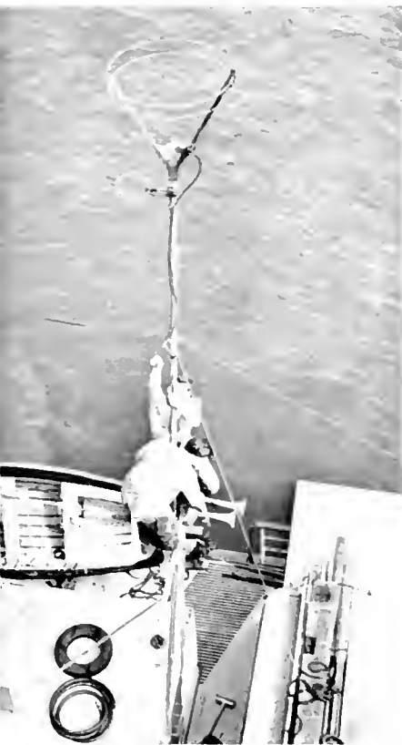
RCA TECHNICIANS ERECTING THE TELEVISION ANTENNA ABOARD THE PILOT BOAT NEW JERSEY. THE SMALL LOOP BELOW THE LARGE ANTENNA IS FOR STATIONS ON CHANNELS 7 TO 13.
