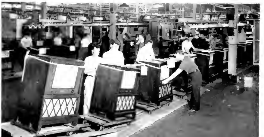
CABINETS FOR TABLE MODELS OF TELEVISION RECEIVERS (ABOVE) MOVE IN A CONTINUOUS LINE AT RCA'S CAMDEN PLANT, WHILE COMPLETED 16-INCH TELEVISION CONSOLES (BELOW) RECEIVE FINAL ADJUSTMENTS AT THE COMPANY'S INDIANAPOLIS FACTORY.
