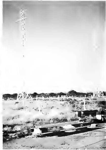
MODERN TOWERS ARE PART OF THE ANTENNA SYSTEM INSTALLED BY THE RADIO CLUB OF MOZAMBIQUE.
