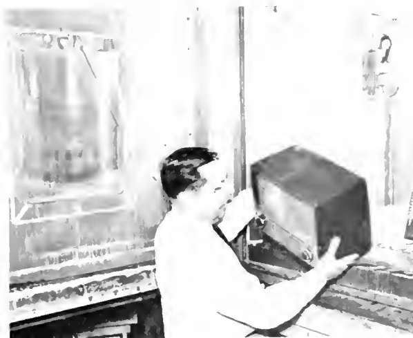
REMOVING AN RCA EXPORT RADIO SET FROM A "TORTURE CHAMBER" WHERE IT HAS BEEN SUBMITTED TO CONDITIONS MORE SEVERE THAN WOULD BE ENCOUNTERED IN THE TROPICS.
