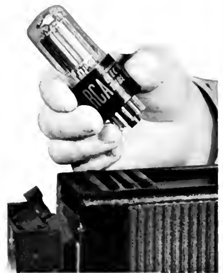
THIS TINY RCA PHOTOTUBE TRANSFORMS LIGHT VARIATIONS OF ULTRAFAX MESSAGES INTO RADIO SIGNALS.
