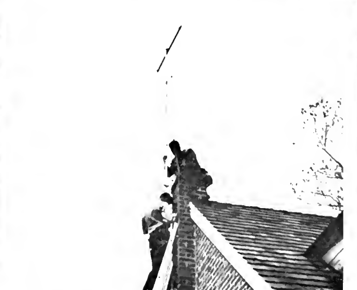
5. Using special rigging and supports, the antenna is clamped securely to the most suitable spot on the roof.
