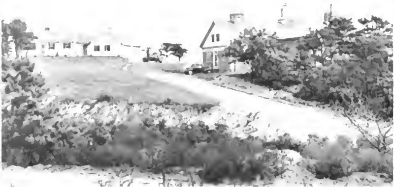
New transmitter building (right) and cottage occupied by engineer in-charge.
