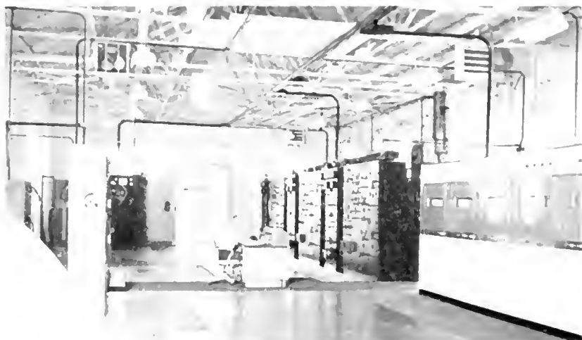
Interior of transmitter building showing high-frequency transmitters, in rear, and 500-kc transmitter (right). Frank Kremp, engineer-in-charge, at console.
