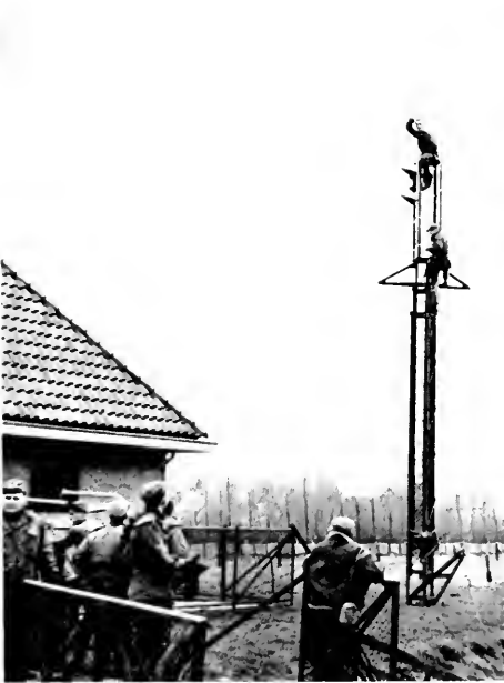
G.I.'s erect emergency microwave tower near Rotterdam to supply communications over Holland's flooded areas.
