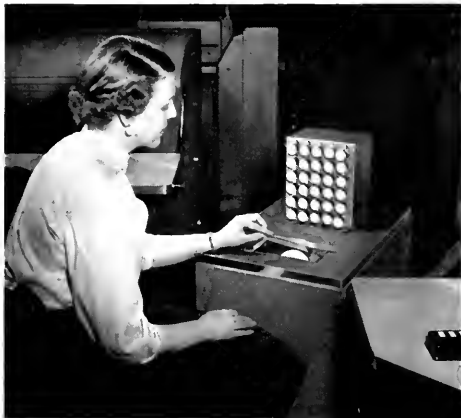
Largest installation yet of "TV Eye" helps to speed banking operations at the Provident Institution for Savings in Boston. File clerk, above, holds signature cord before the camera for viewing by teller, right.
