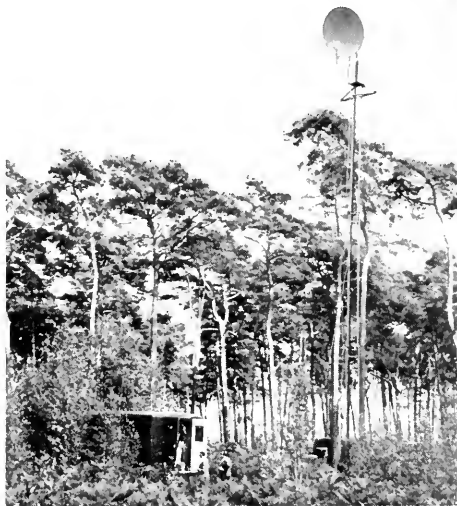
This microwave antenna, located at a secluded operations base in Western Europe, is one of the links in an RCA radio network linking Allied air installations with Central Europe headquarters of the U. S. Air Force.
