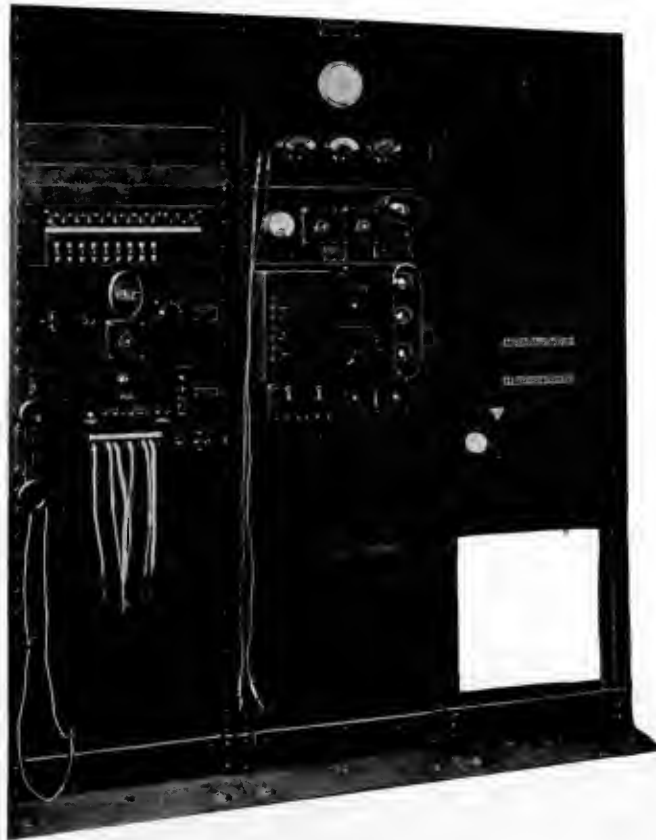
CONTROL EQUIPMENT OF THE PRAGUE, CZECHO-SLOVAKIA STATION
