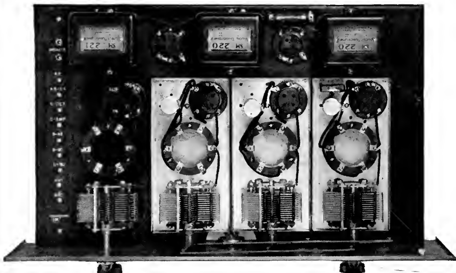
PREPARATORY TO PLACING THE STAGE SHIELDS IN POSITION
