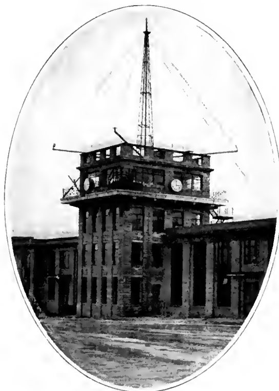
The radio control room is located on the top floor of the tower of the Terminal Building at the Croydon Air Port. On the top of the tower are the directional antennas and a 100-foot horizontal antenna.
