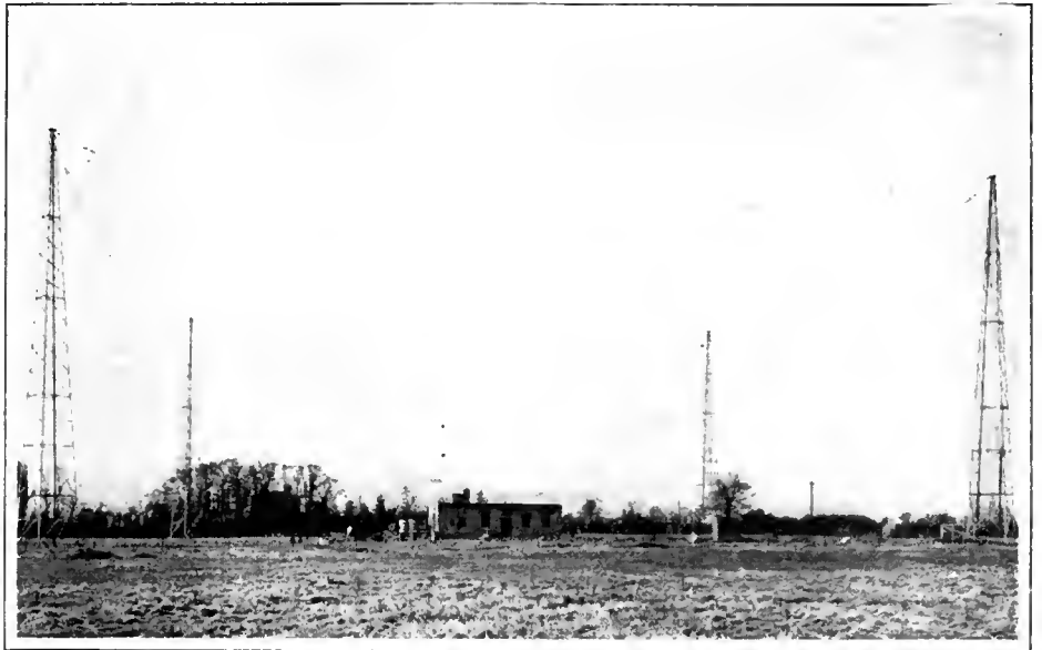
The four transmitters and antenna system are located 4½ miles from the flying field, leaving the field itself clear for taking off and landing. The antenna masts, placed at the corners of a 250-foot square, are 100 feet in height, and support four cage aerials of the inverted "L" type
