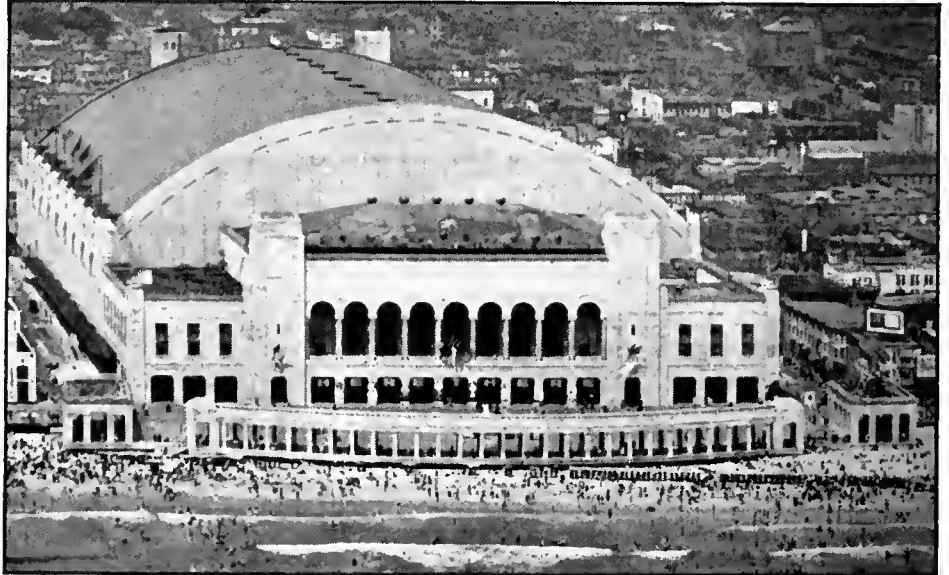
The new mammoth $15,000,000 civic auditorium on the boardwalk at Atlantic City where the Annual Convention and Trade Show of the Radio Manufacturers' Association will be held during the week of June 2. The building is the last word in convention hall construction. It is 350 feet wide by 650 feet deep and provides 85,000 sq. ft. of exhibition space.
