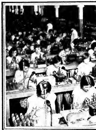
General view of assembly floor where vacuum tubes are mounted.
