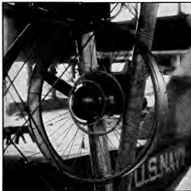
View of a wind-driven motor generator.
