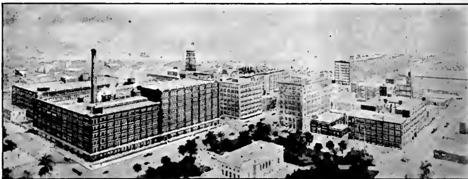
General view of the plant of the Victor Talking Machine Division of the Radio-Victor Corporation of America.
