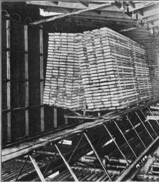
Interior of Humidity Controlled Dry Kiln
