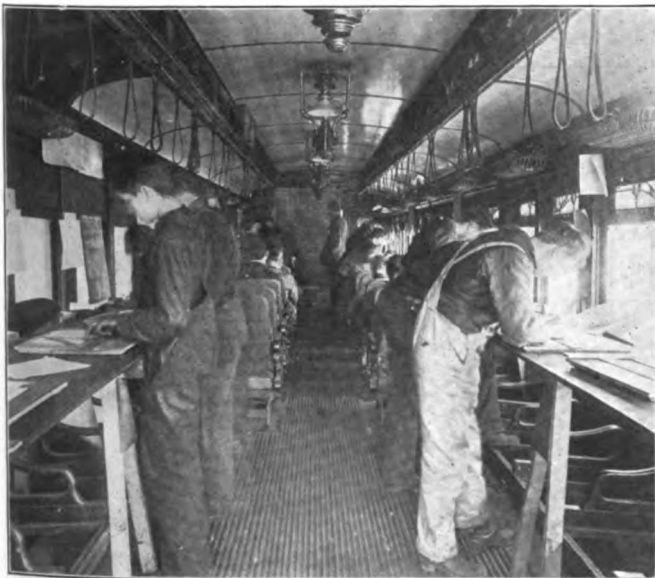
Interior of Staten Island Apprentice School Car
