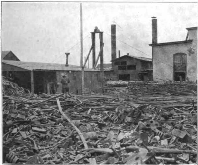
Fig. 1—Scrap Pile at St. Cloud
