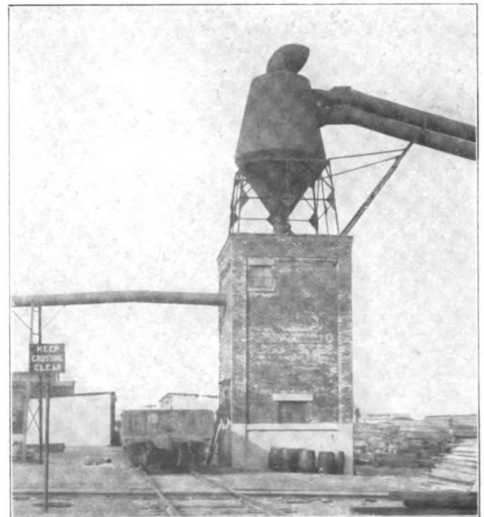
Sawdust House and Separator for Planing Mill
