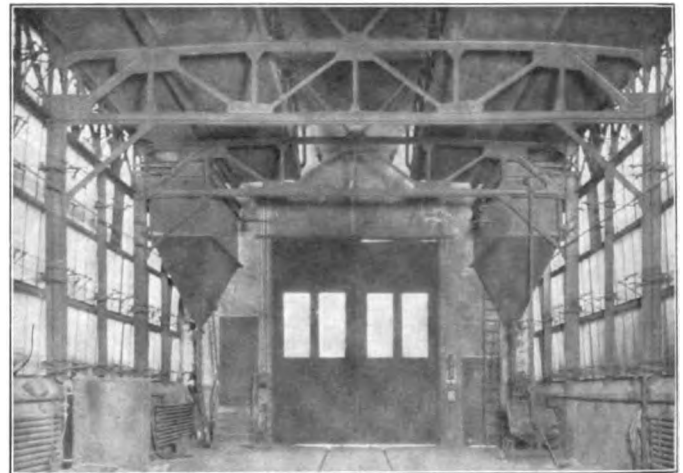
Interior of the Sand Blast House Showing the Dry Sand Storage Bins
