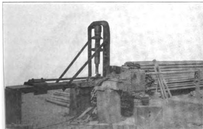
Fig. 5—Outdoor Welding Machine and Furnace for Piecing Short Tubes
