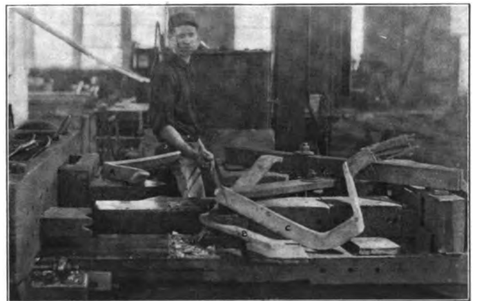
Fig. 14—Formers for Making Brake Mast Supports
