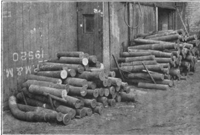
Fig. 4—Sheared Wrought Iron Axles Which Are to be Rolled Into Refined Iron Bars
