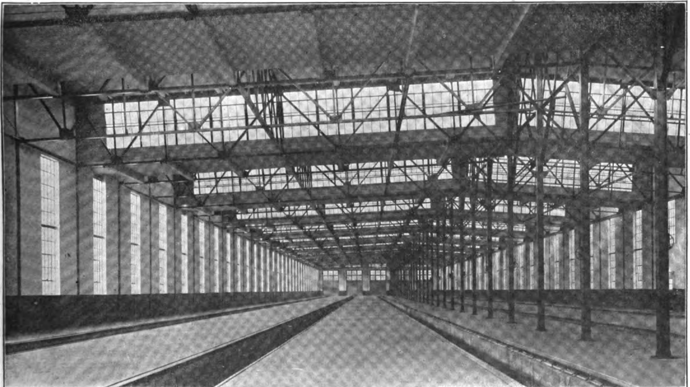
Interior of the Longitudinal Type Shop
