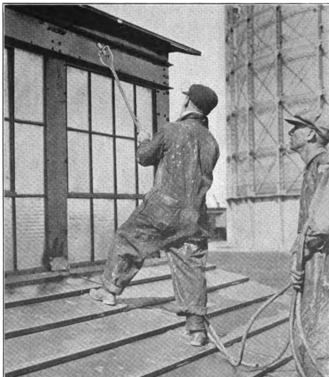
Vortex Painter in Use On Metal Building
