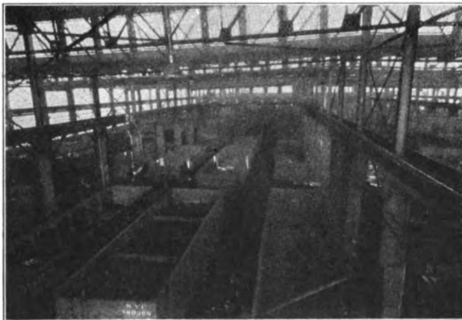
One of the Erecting Bays
