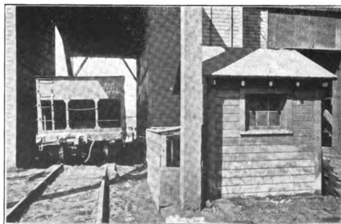
Fig. 2. Car Hauling Winch Installed at Coaling Station
