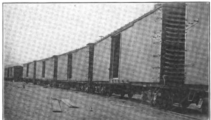
Fig. 2—A String of Steel Underframe Cars After Rebuilding
