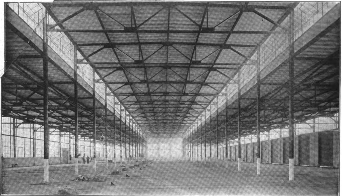
Interior View of the Transverse Shop
