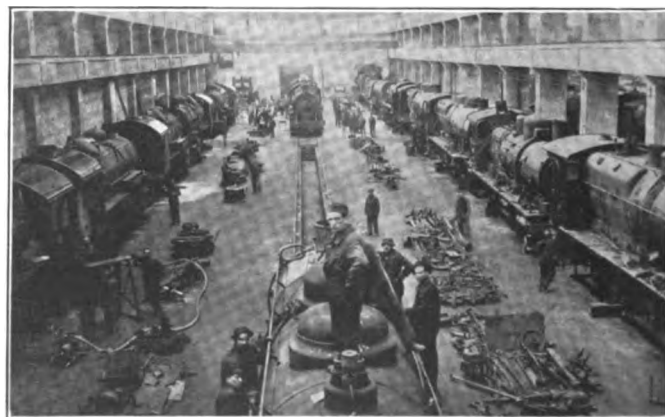
One of the Two Bays of the Erecting Shop of the A. E. F. Engineers at Nevers, France. American Locomotives on the Left and Centre Tracks. French Locomotives on the Right Hand Track.
