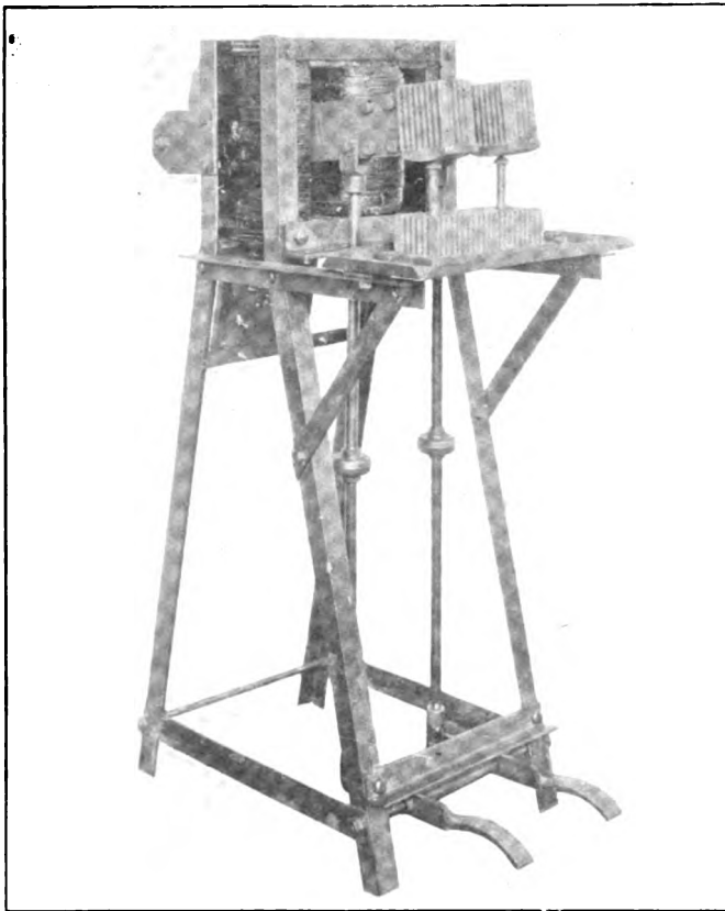
A Two-Head General Electric Rivet Heater
