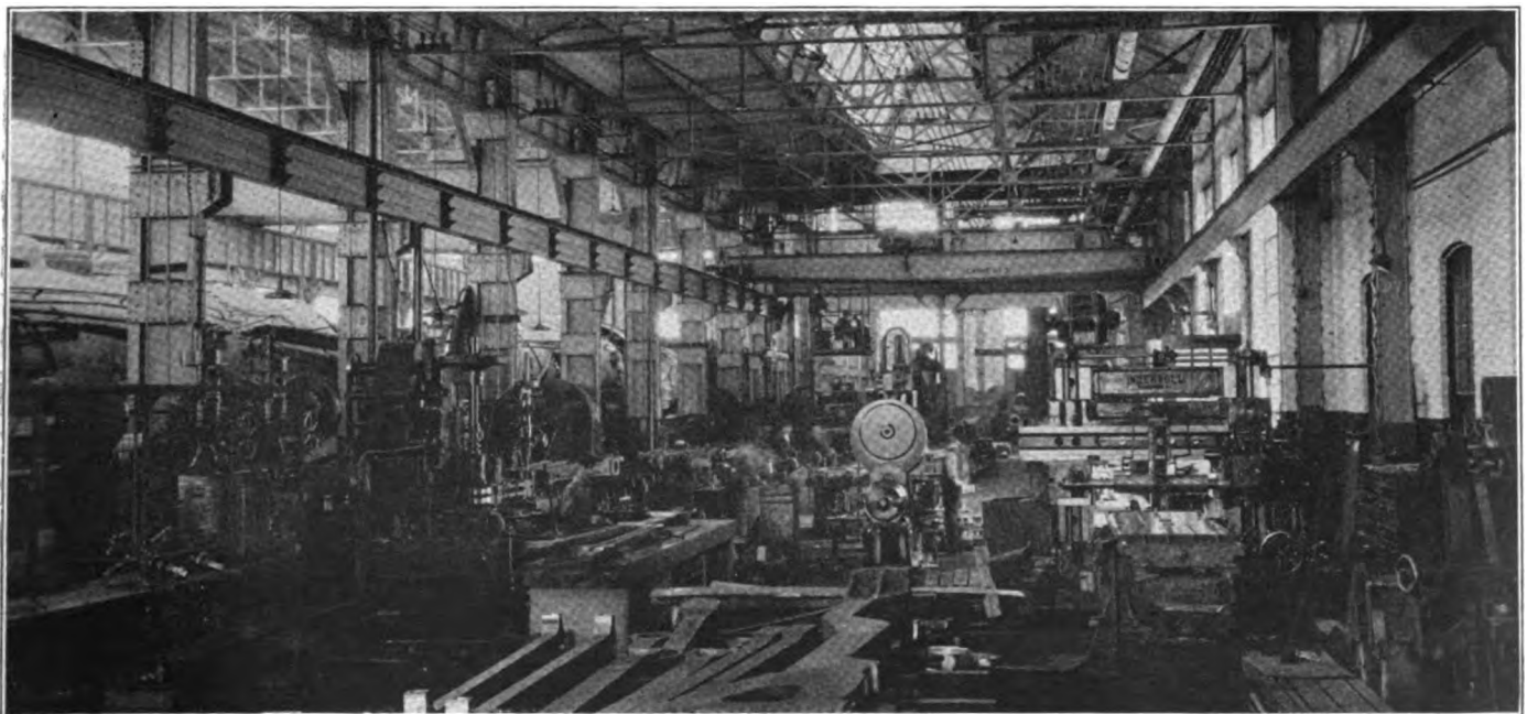
Heavy Machine Bay in the Erecting Shop
