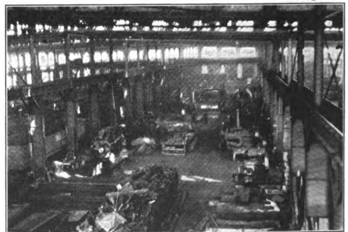
Looking Down Central Machine Bay
