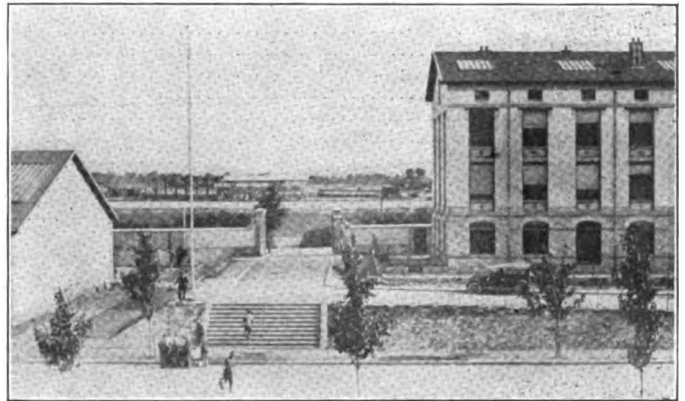
Administration Building and Entrance to Shops
