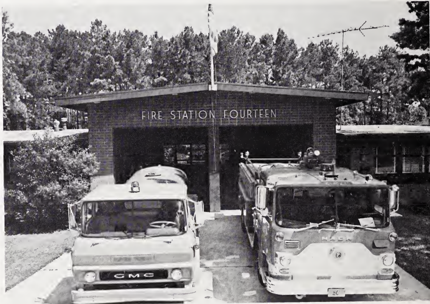
Fire Station Fourteen — 4220 Lake Boone Trail
