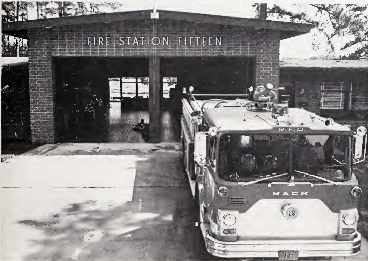
Fire Station Fifteen — 1815 Spring Forest Road
