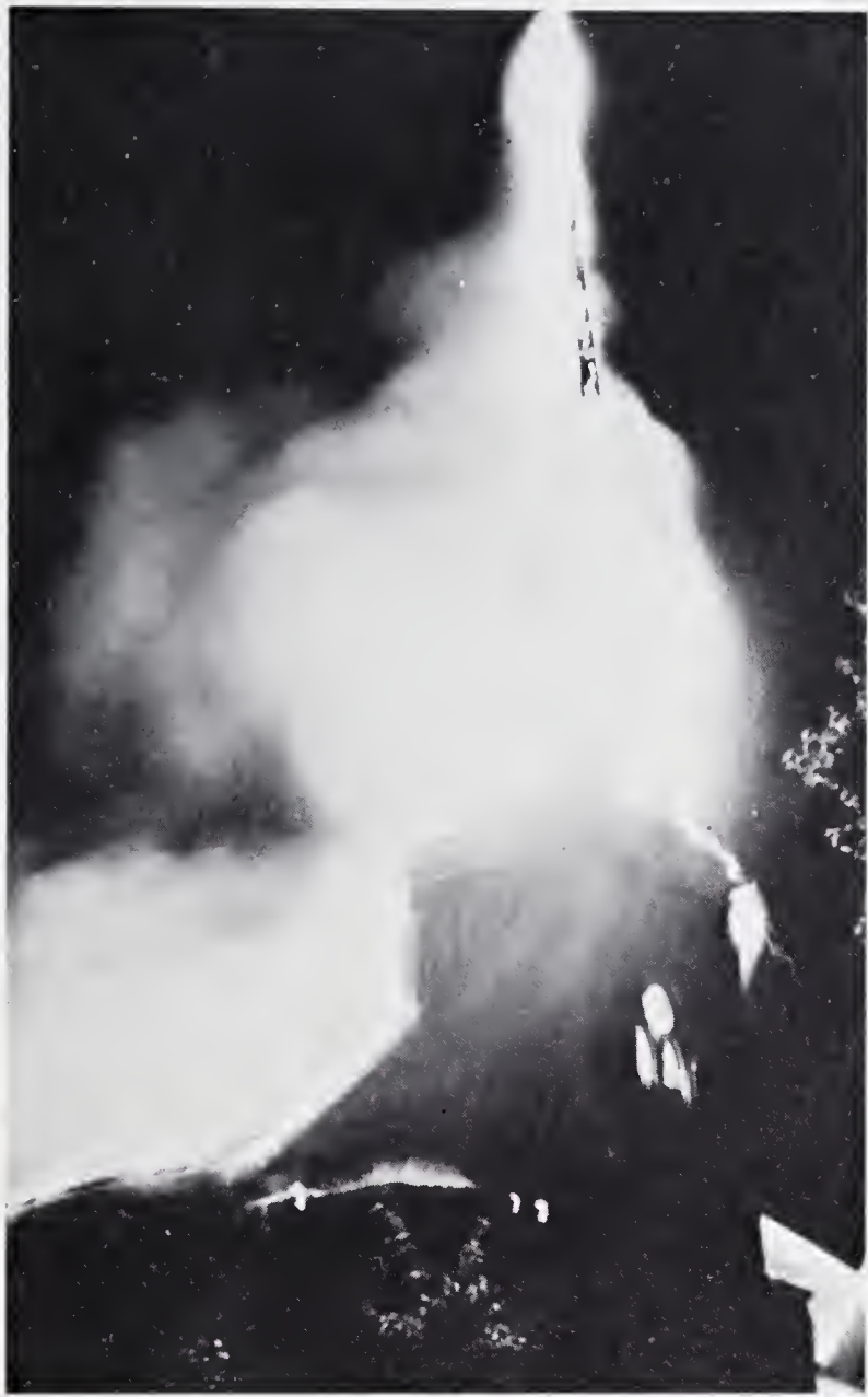
Edenton Street Church Steeple Ablaze
