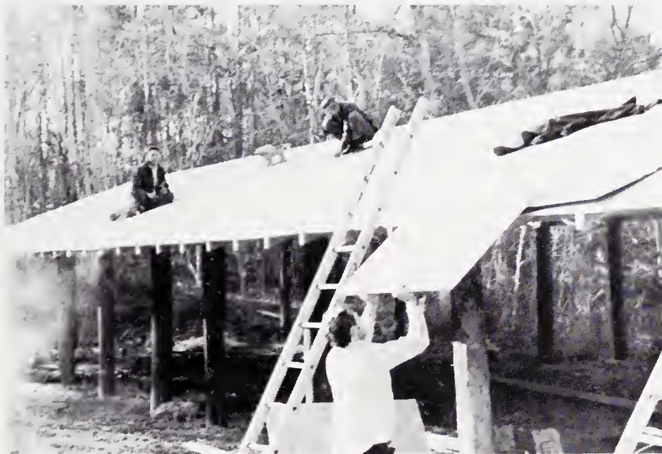
Construction of Picnic Shelter
