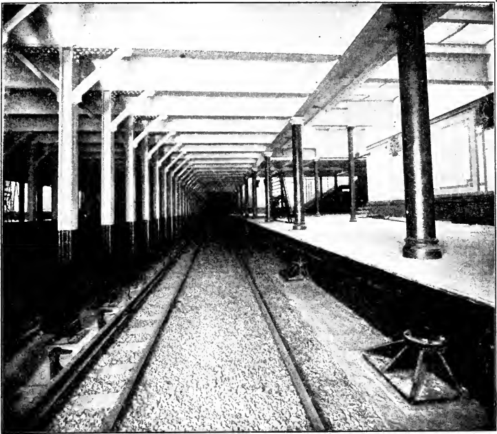
EIGHTEENTH STREET STATION — Showing concrete and steel construction.
