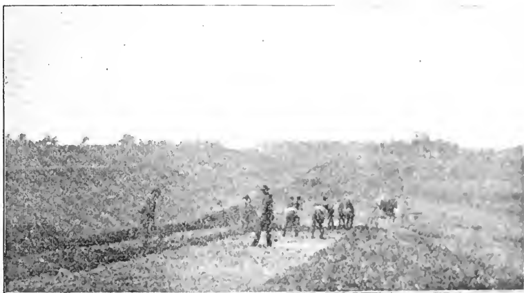
CONVICTS PREPARING MACADAM IN RALEIGH TOWNSHIP.
