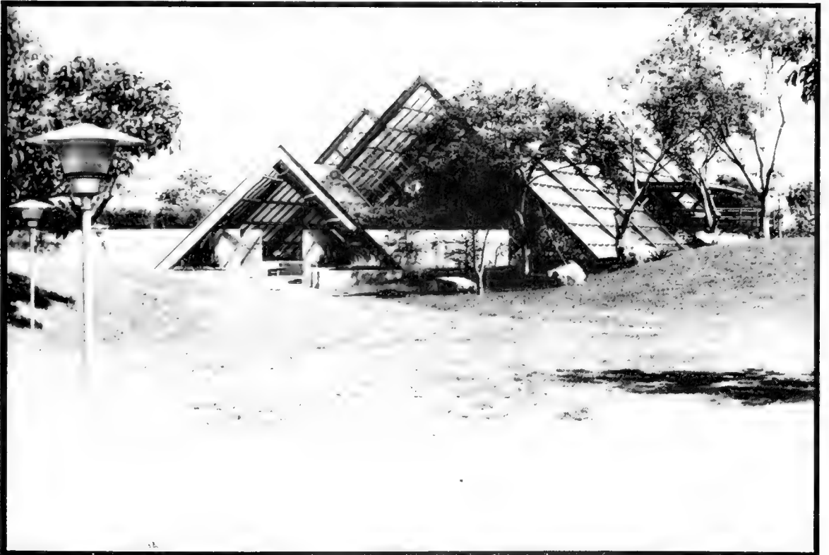
Figure 5 : A partial view of the new complex of display pavilions
