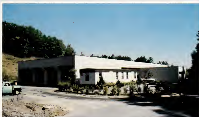
In the Power Mechanics Building students take classes in the Diesel and Equipment Technology and Automotive Mechanics Program.
