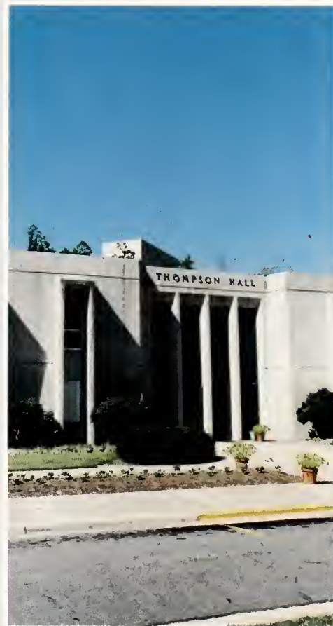
Thompson Hall houses the Library, Administrative Offices, Commons, and the Business Department.
