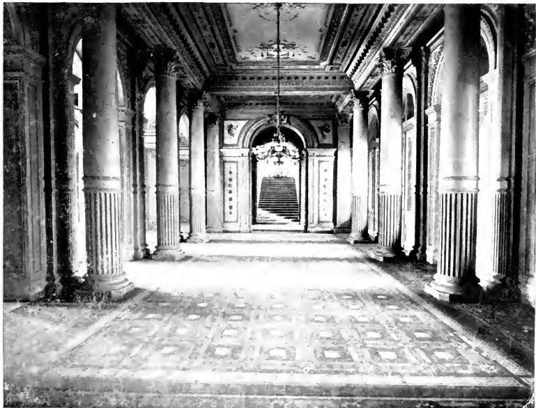
EXTERIOR AND INTERIOR OF THE "CASA ROSADA."
