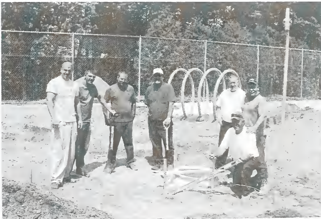
Parks & Recreation Dept. & DPW employees installing the new splash pad at the Rec. pool on Hampton Road. L-R: Mike Gingras, Brian Shea, Wayne Almon, Jim Colbert, Justin Hall, Steve Tucker, Dick Rowe
