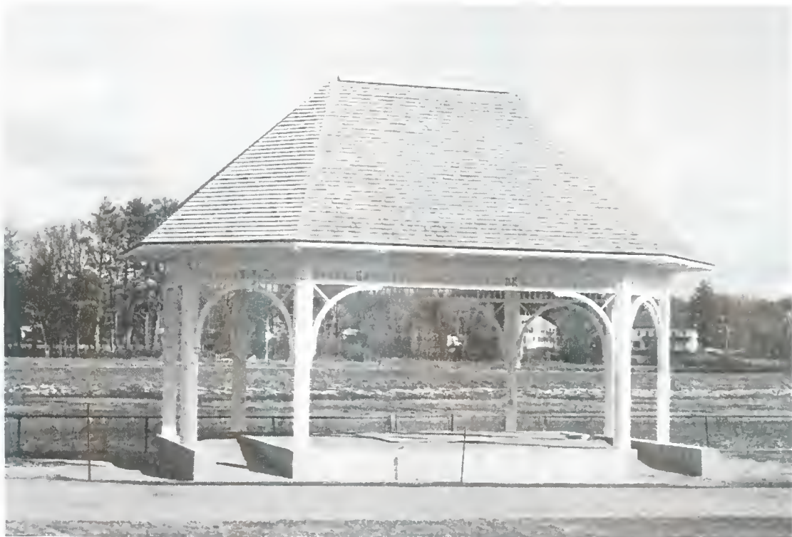
The new Pavillion at Swasey Parkway, still under construction
