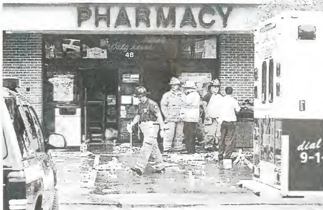
Walgreen's roof collapse during hail storm – July 2006
