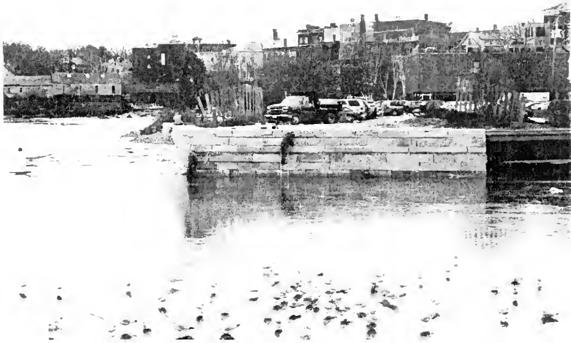
New seawall at Stewart Park
