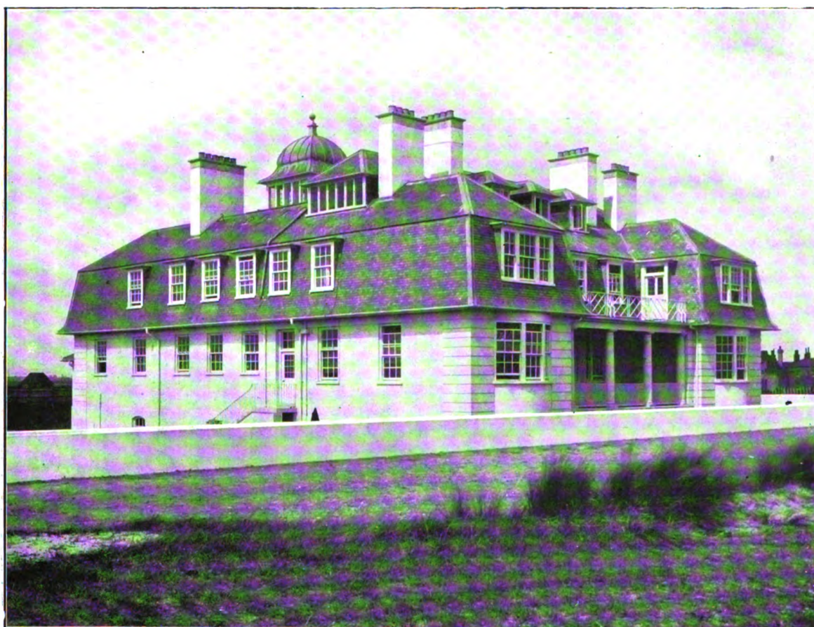
The walls are built with a hollow space, and are "harled" or rough-casted outside. The roofs are covered with Delabole slates.
