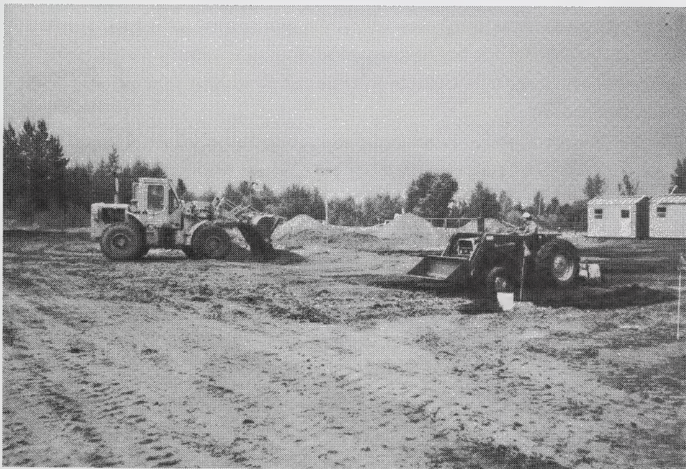
Figure 13. Replacing the top 15 cm of soil with the loader (right)
