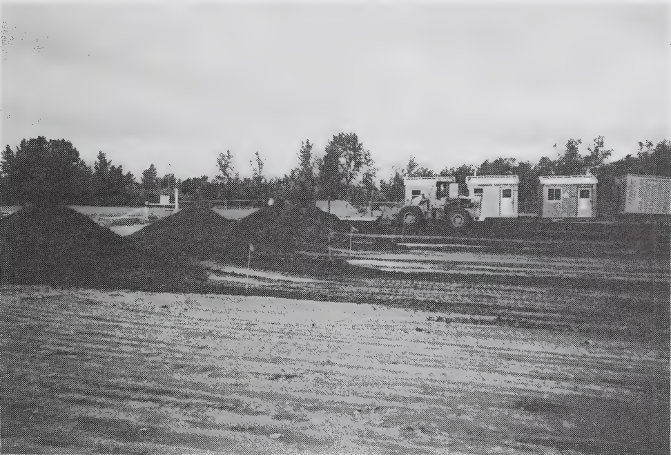
Figure 12. Stripping the top 15 cm of soil at Devon by block.
