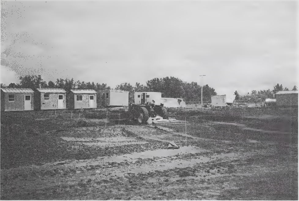
Figure 11. Rotovating the 15 to 30 cm soil depth at Devon.
