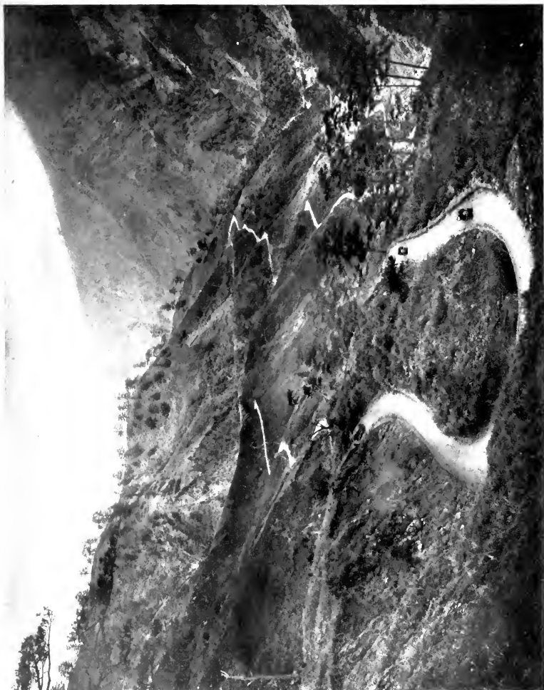
THE ZIGZAG. HOW THE BENGUET ROAD CLIMBS TO AN ALTITUDE OF OVER 5,000 FEET IN SIX MILES
