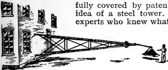
Testing the Towers.
