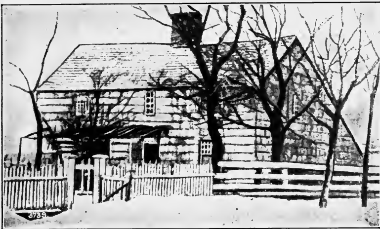
THOMAS SAYRE — ERECTED IN 1648 — DEMOLISHED IN 1912 — SOUTHAMPTON, L. I. (Howell and Fordham, Southampton)
