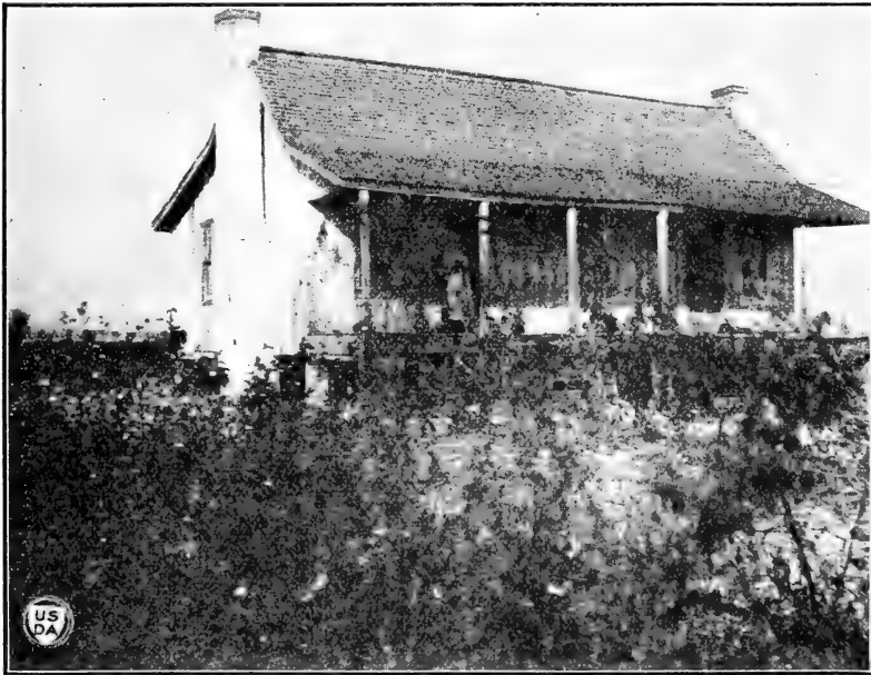
FIG. 13.—The small one to two room labor cabins on the plantation are gradually being displaced by comfortable dwellings. Upper: Three-room, "shotgun" type. Lower: Four-room, double chimney type. Both are considered desirable in economy of construction, comfort, and ventilation.
