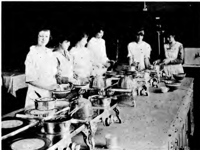
NEW ELECTRICAL EQUIPMENT, B. Y. U.
