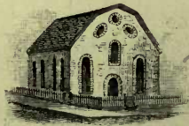
LUTHERAN CHURCH, CORNER WILLIAM AND FRANKFORT STREETS
