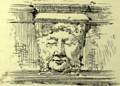
HEAD OVER WINDOW IN WALTON HOUSE
