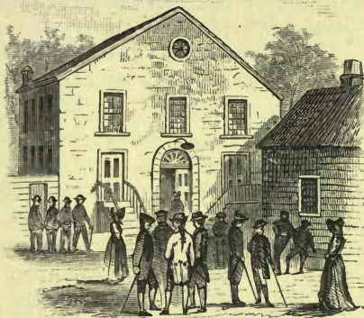
METHODIST CHURCH, JOHN STREET. 1768
