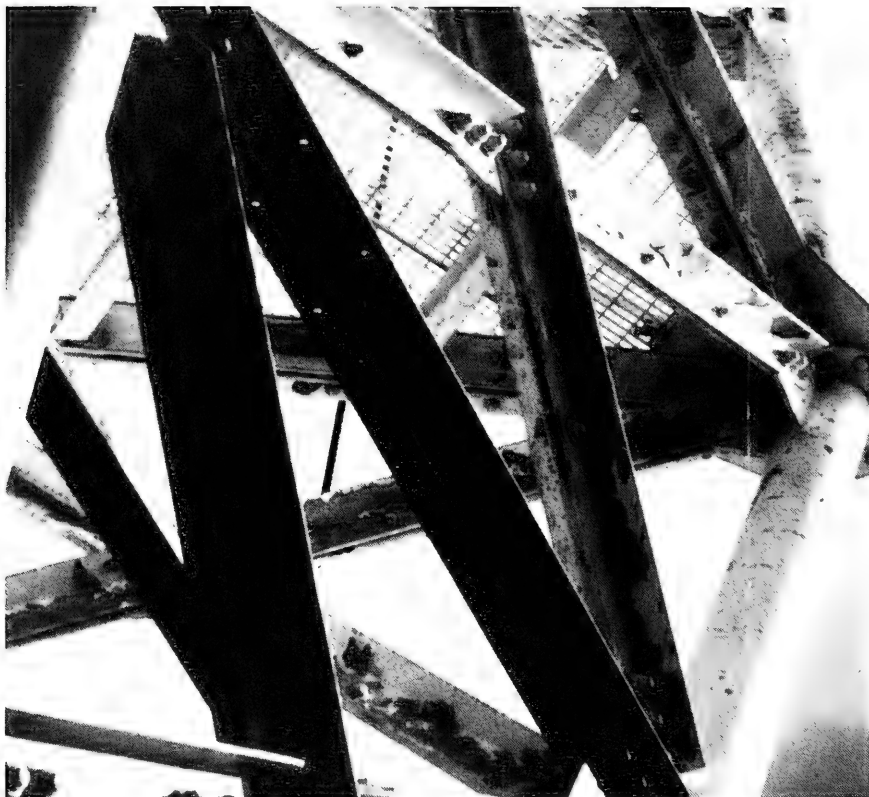
Figure 5. Paint peeling from galvanized steel.
