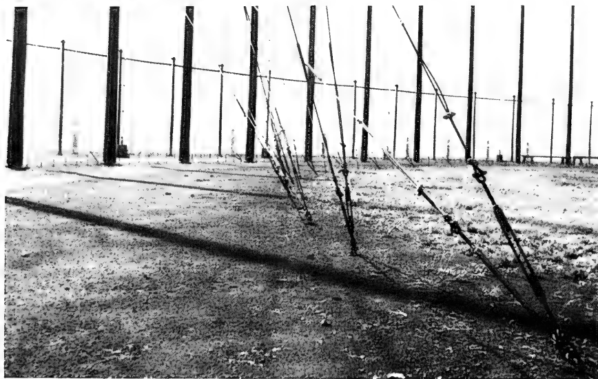
Figure 14. Glass-reinforced plastic guy line with dampener.
