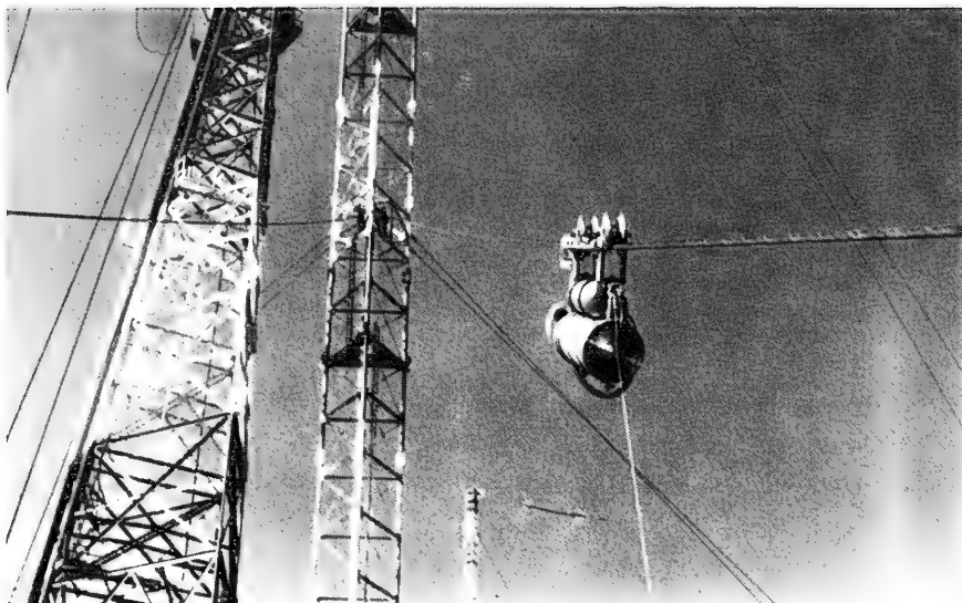
Figure 13. Equipment ascending guy line.
