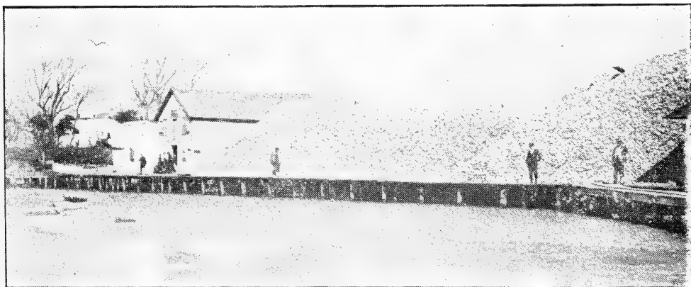
WASTE PLACES BUILT UP BY OYSTER TRADE The fifty thousand bushels of shells will be sowed to catch spawn
