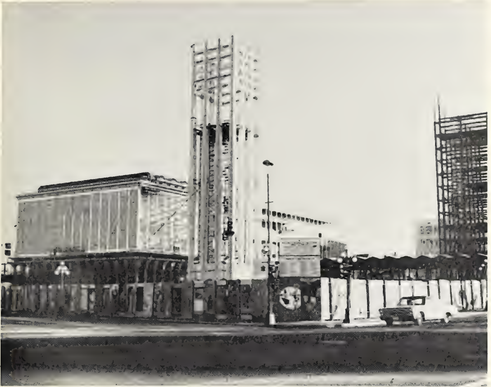
British Columbia Provincial Museum and Archives complex with Carillon Tower in foreground, as it looked in November, 1967.
