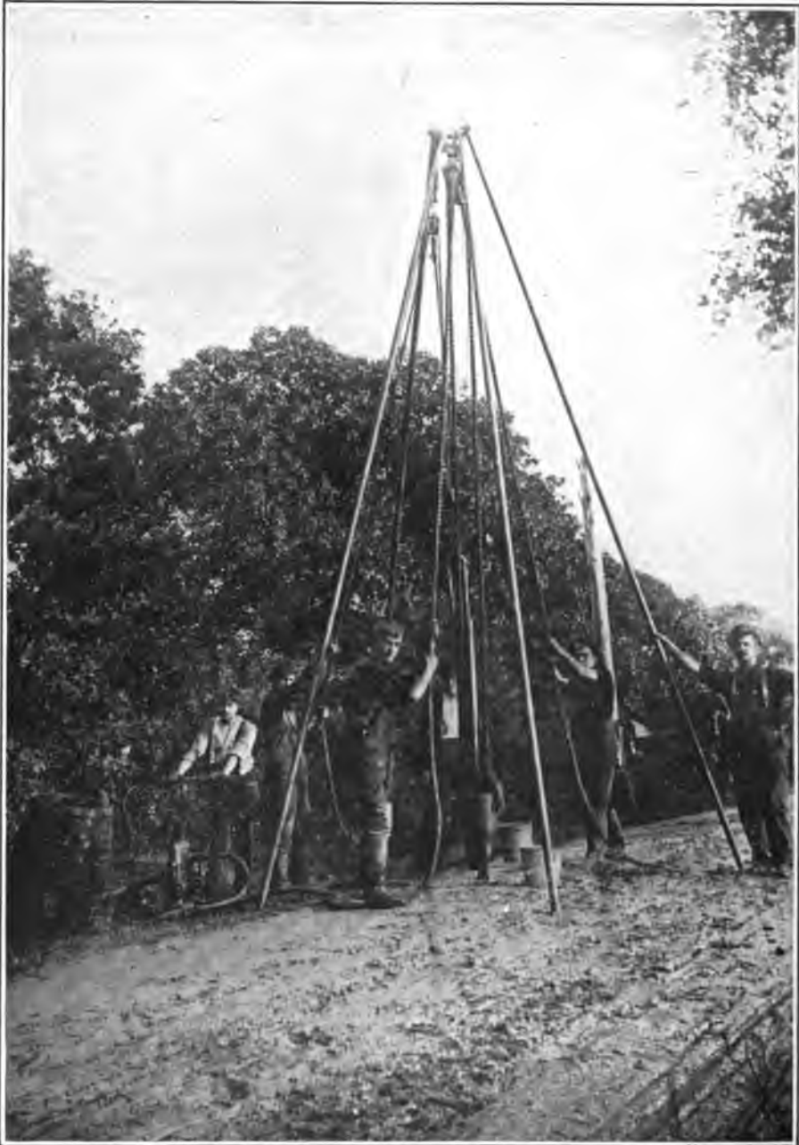
RIG ARRANGED BY THE COMMISSION.
