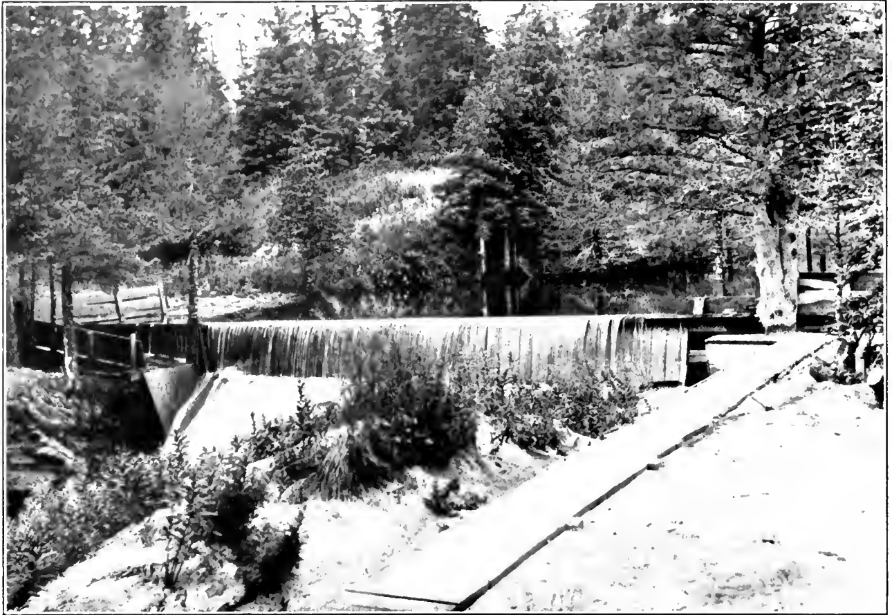
WATER-SUPPLY RESERVOIR AT AFOGNAK HATCHERY.
