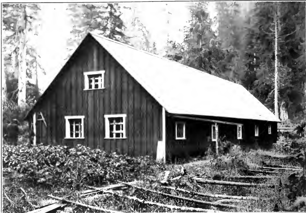
HATCHERY BUILDING, BOCA DE QUADRA.
