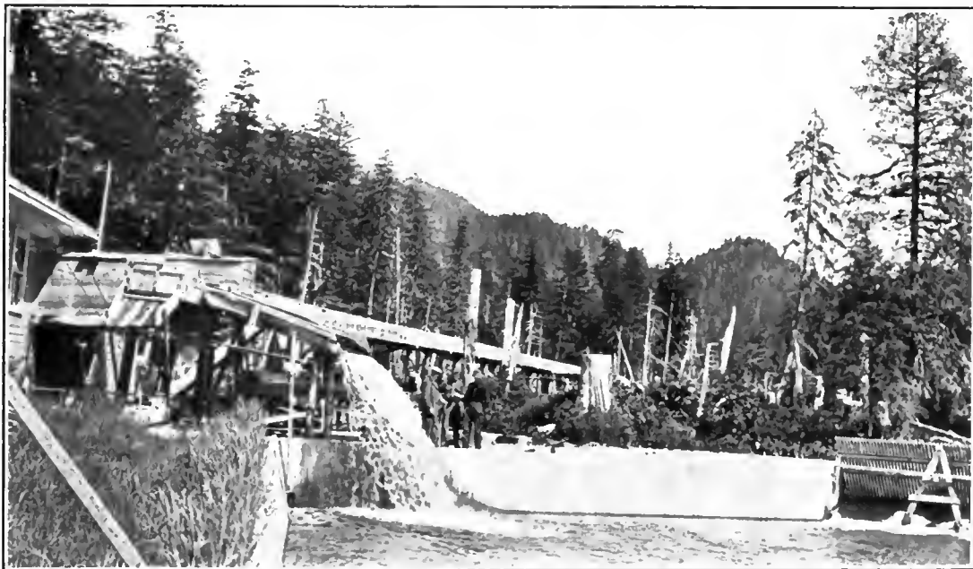
INTAKE OF WATER-SUPPLY FLUME AT YES BAY HATCHERY.
