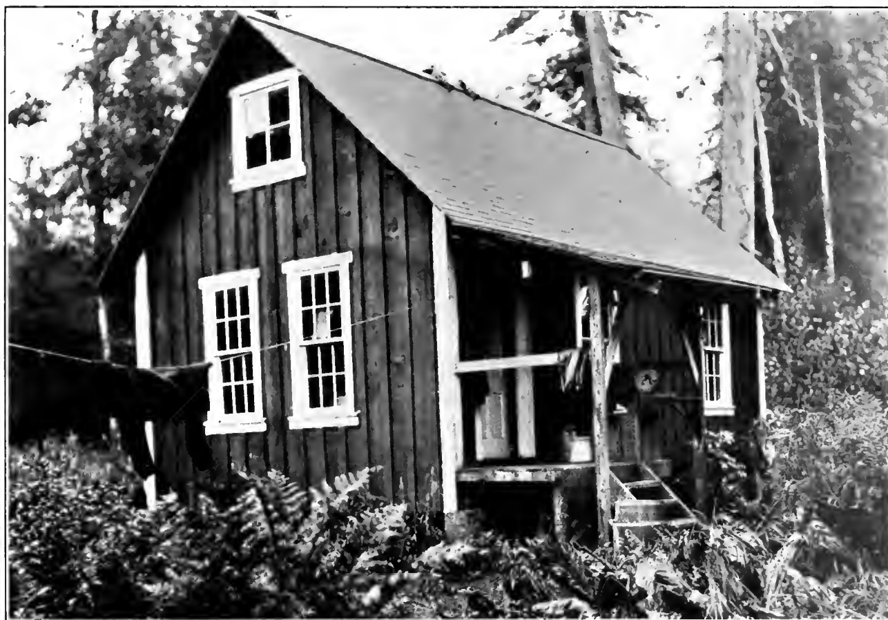
LIVING QUARTERS, BOCA DE QUADRA HATCHERY.
