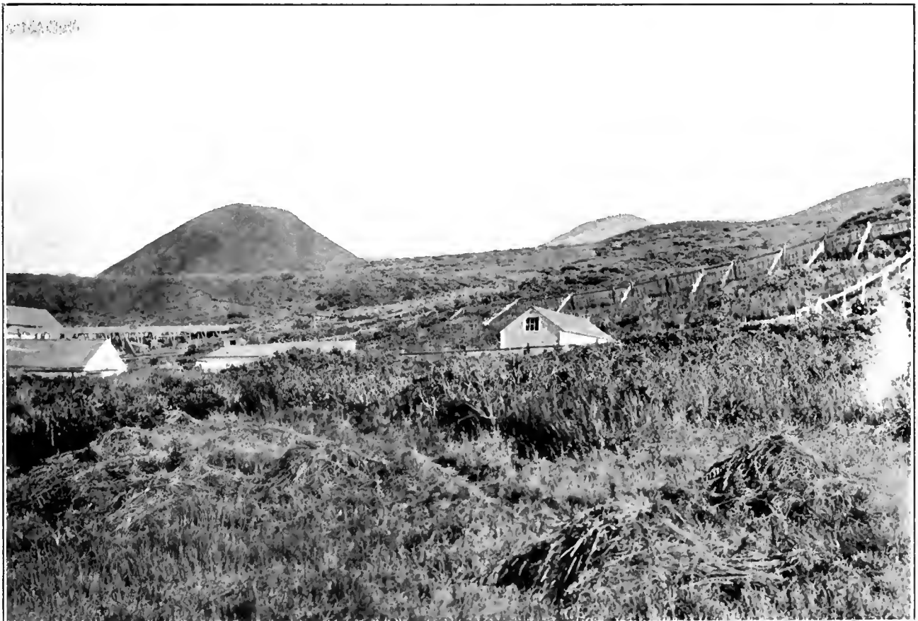
KARLUK HATCHERY SHOWING WATER SUPPLY AND TRAMWAY FOR HANDLING ADULT BREEDING SALMON AND FRY.
