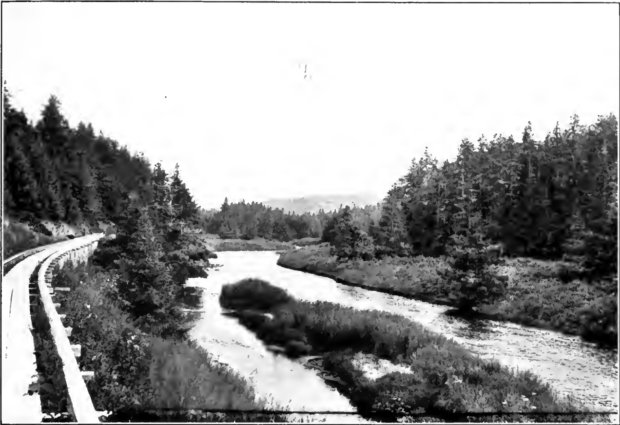
TRAMWAY LEADING FROM SALT WATER TO AFOGNAK HATCHERY, SHOWING ALSO LITNIK RIVER.
