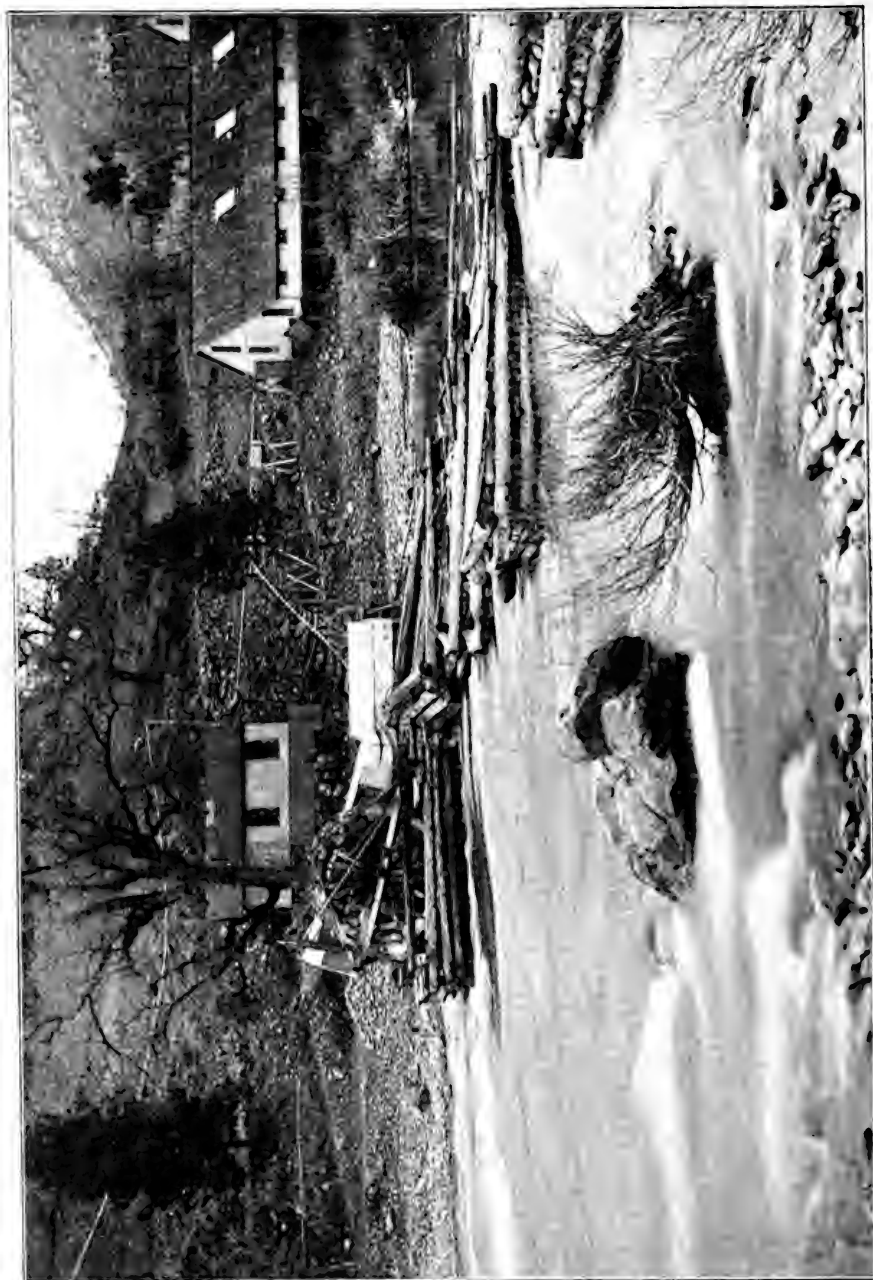
ENGINE-HOUSE AND HATCHERY, BAIRD; CURRENT-WHEEL, AND PIERS FOR HOLDING RACK USED TO STOP ASCENT OF SALMON.
