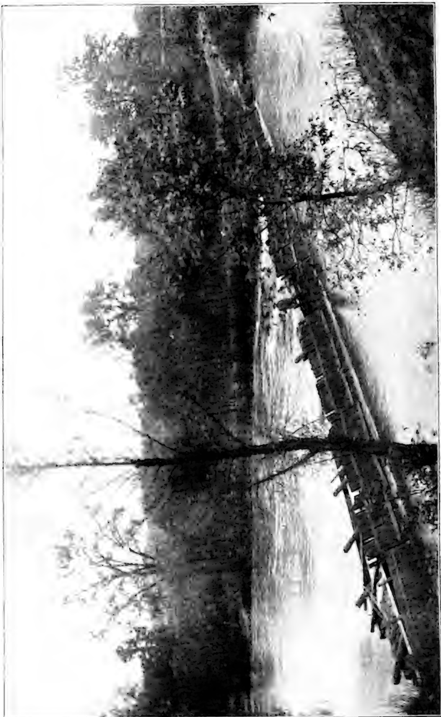
RACK FOR STOPPING ASCENT OF SALMON, AT BATTLE CREEK CALIFORNIA.
