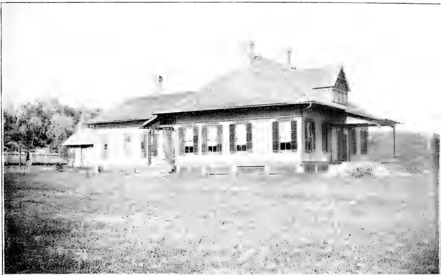
SAN MARCOS STATION TEXAS—WEST SIDE OF SUPERINTENDENT S DWELLING
